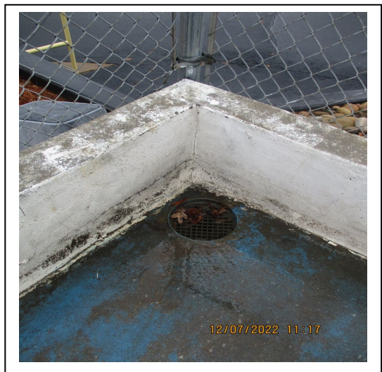
Photo #7 – CAA pad drain. The drain is connected to the stormwater drain (Photo #8).
