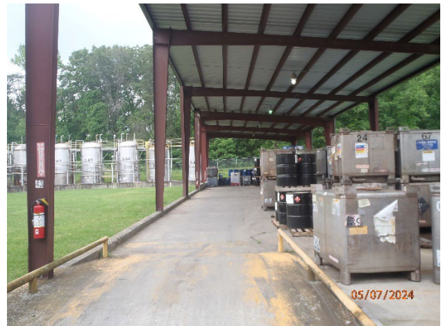
Picture 51 – Flammable Storage
