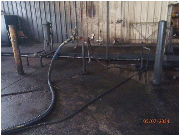
Picture 86 – Building 6 loading area with resin and water on ground
