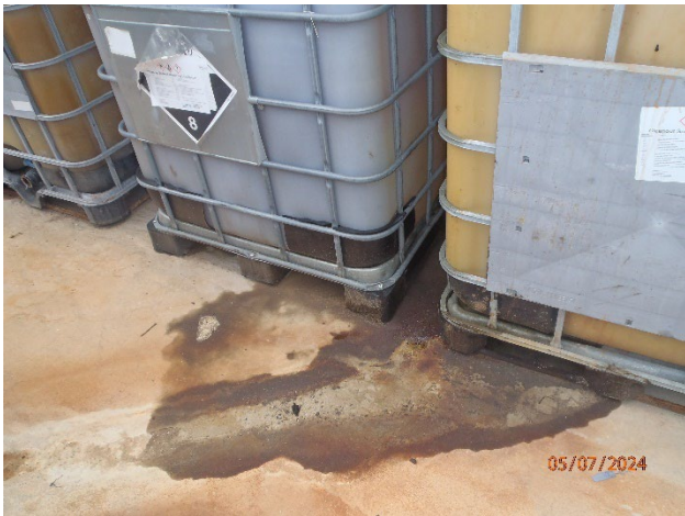
Picture 92 – Tanker Lot with clean out solvent release to ground
