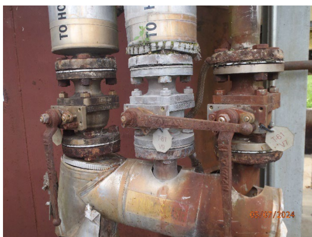
Picture 53 – Hazardous Waste T-61 missing BB tags
