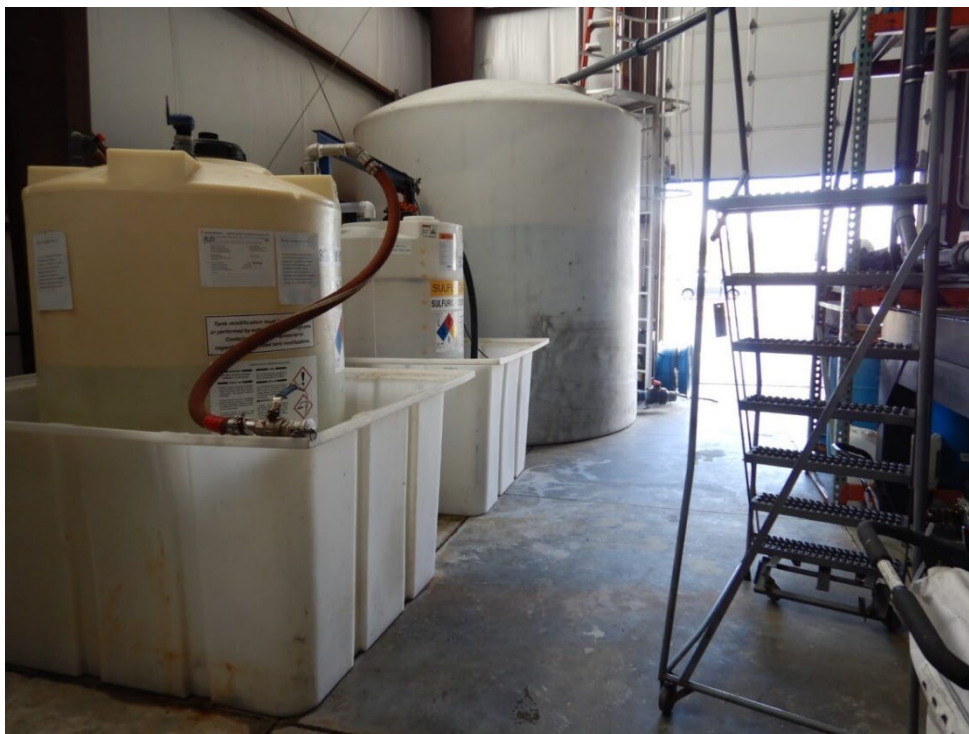
Photograph 1: View of Cargill's sodium hydroxide and sulfuric acid tanks in secondary containment.
