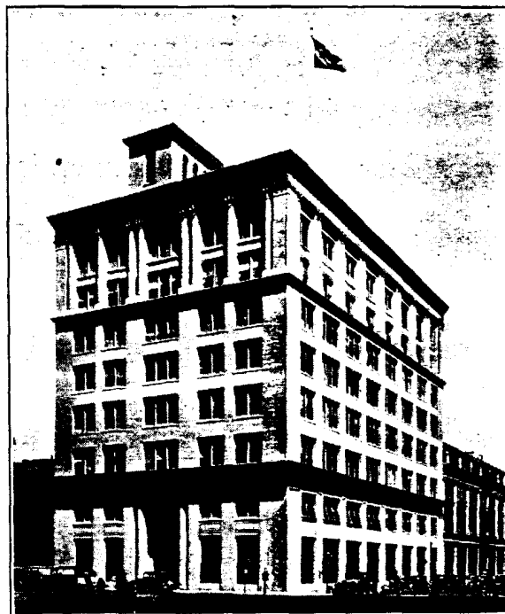
Oceanic Building, San Francisco. The concrete upper stories are made to imitate the two granite lower stories by the use of white lead and granite aggregate.
