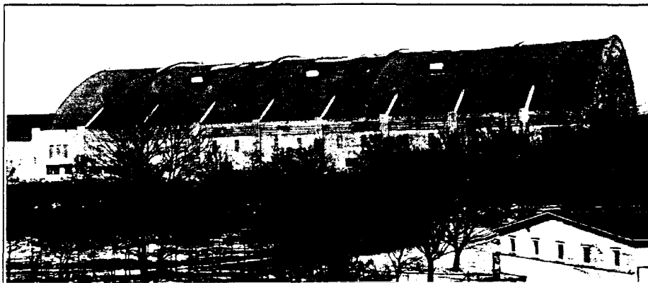
Sports arena at Hershey, Pa., measuring 245½ x 364 ft. over-all. The stiffening arches for the roof rest on lead pads.
