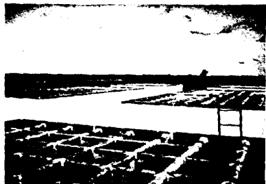
Three views of the "honey comb" acoustical block towers with lead flashing and copings at the Engine Test Building of the Sacramento Air Depot.
