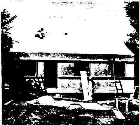
Phenol plywood was used for interior and exterior walls and roof sheathing. Hard sheet lead formed the chimney flashing.
