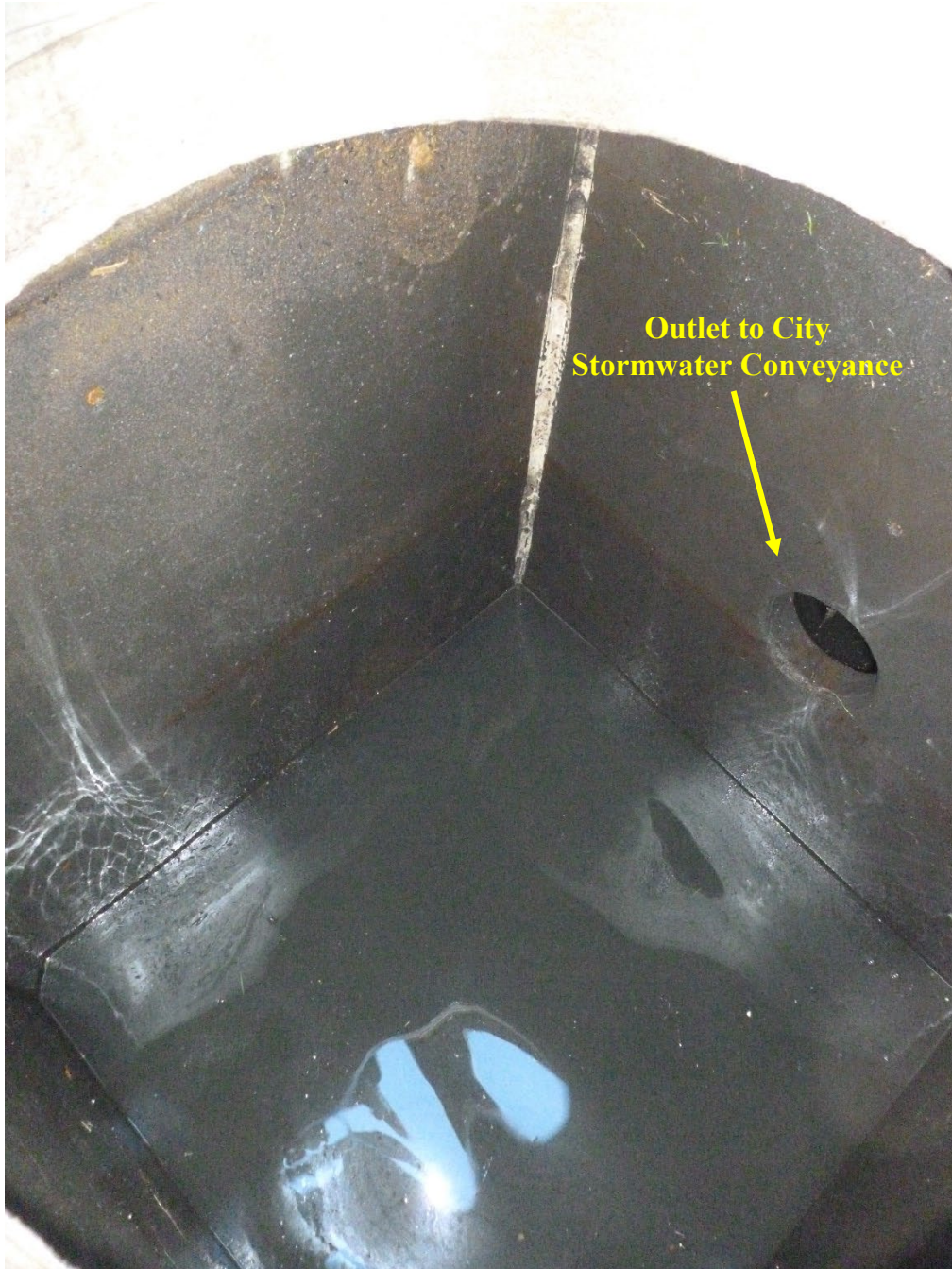
Photo 4 / P1010152 – Catch basin 5 Vault, interior
