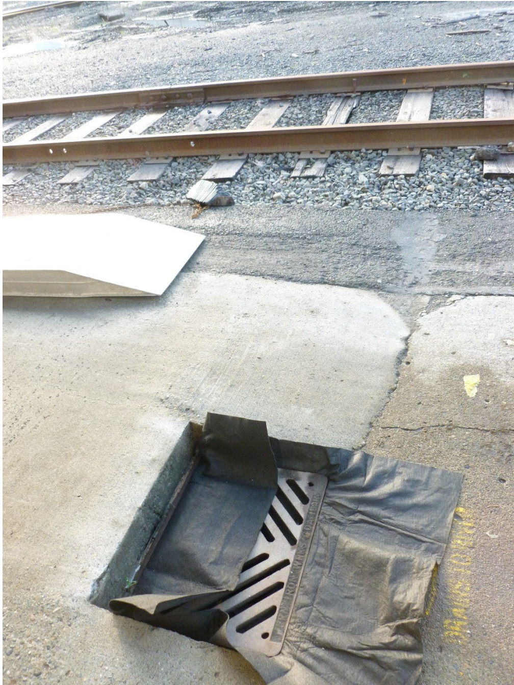
Photo 11 / P1010163 – Catch Basin 3, facing west, close-up
