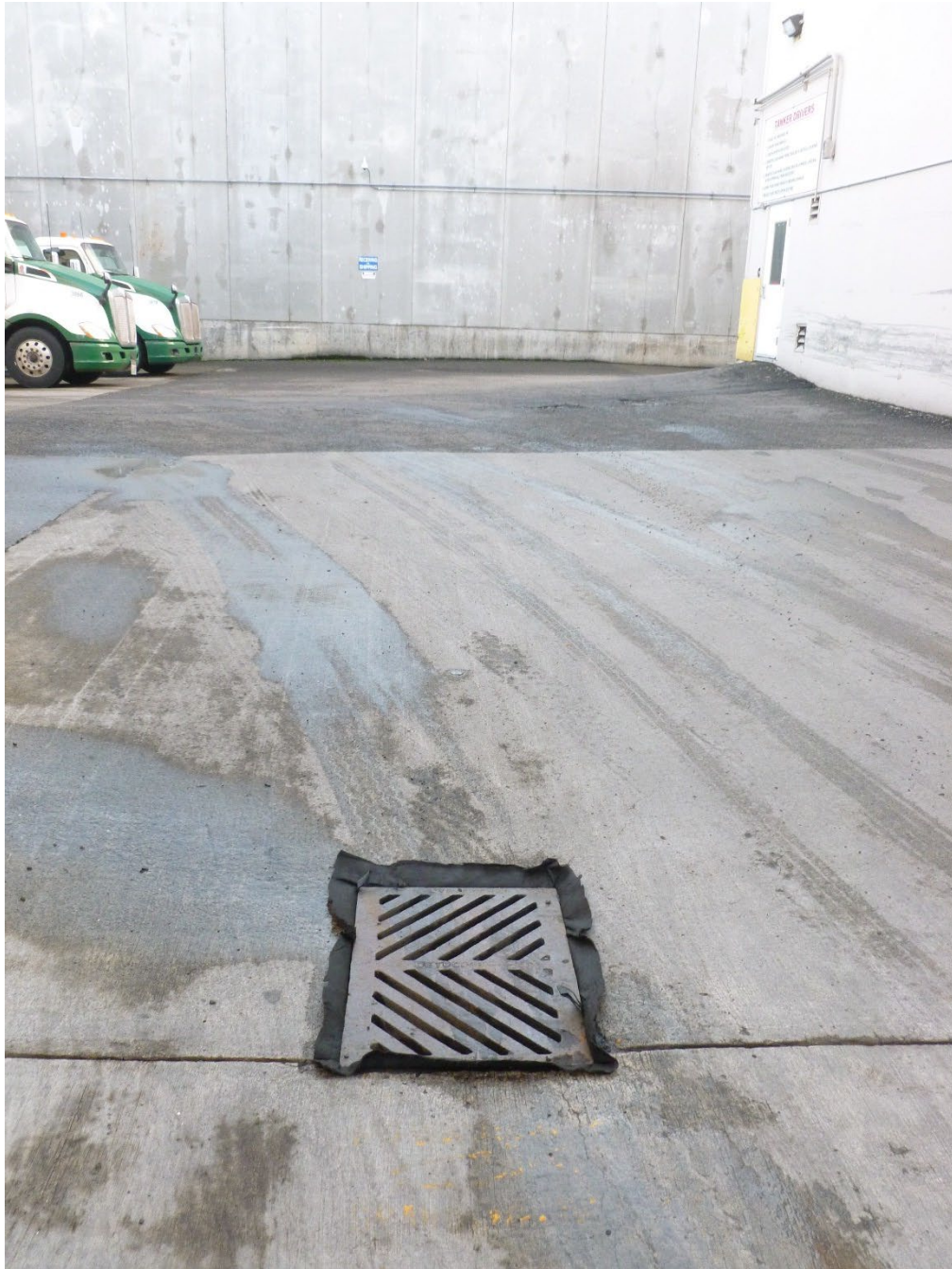
Photo 13 / P1010165 – Catch Basin 2, facing north
