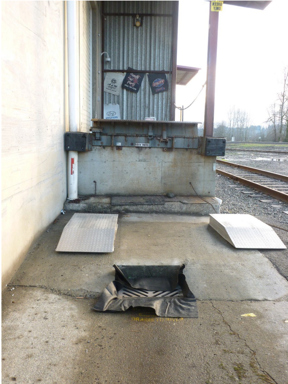
Photo 10 / P1010161 – Catch Basin 3, facing north
