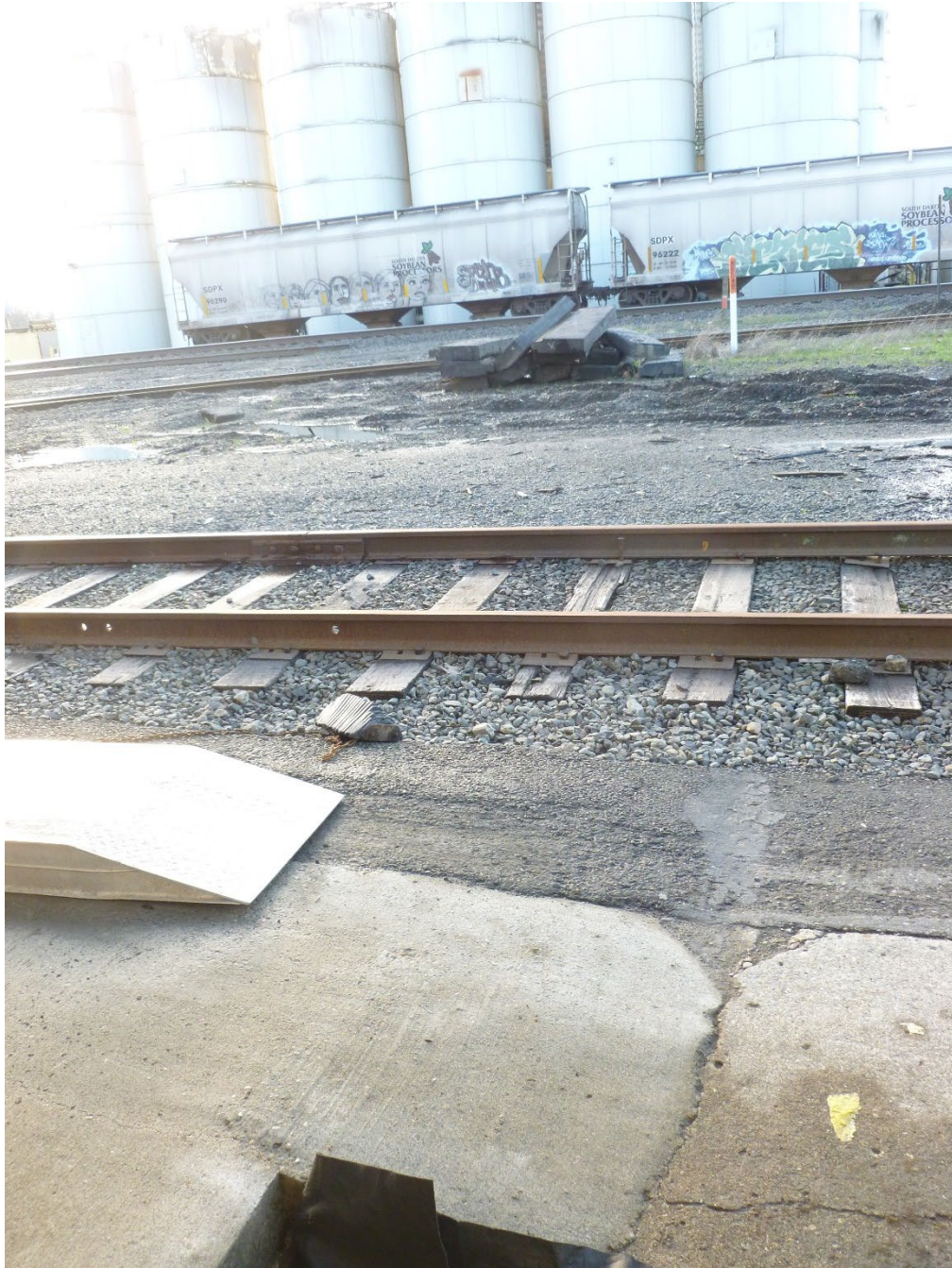
Photo 12 / P1010164 – Catch Basin 3, facing west, extended view
