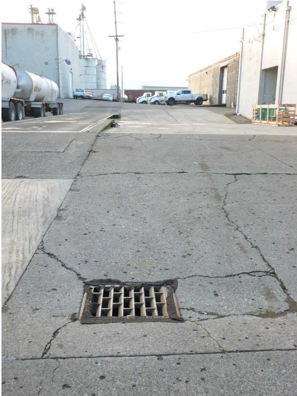
Photo 9 / P1010159 – Catch Basin 8, facing west
