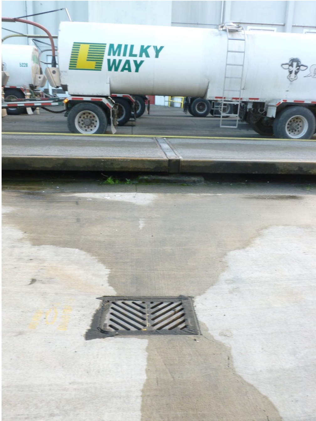
Photo 7 / P1010160 – Catch Basin 4, facing north
