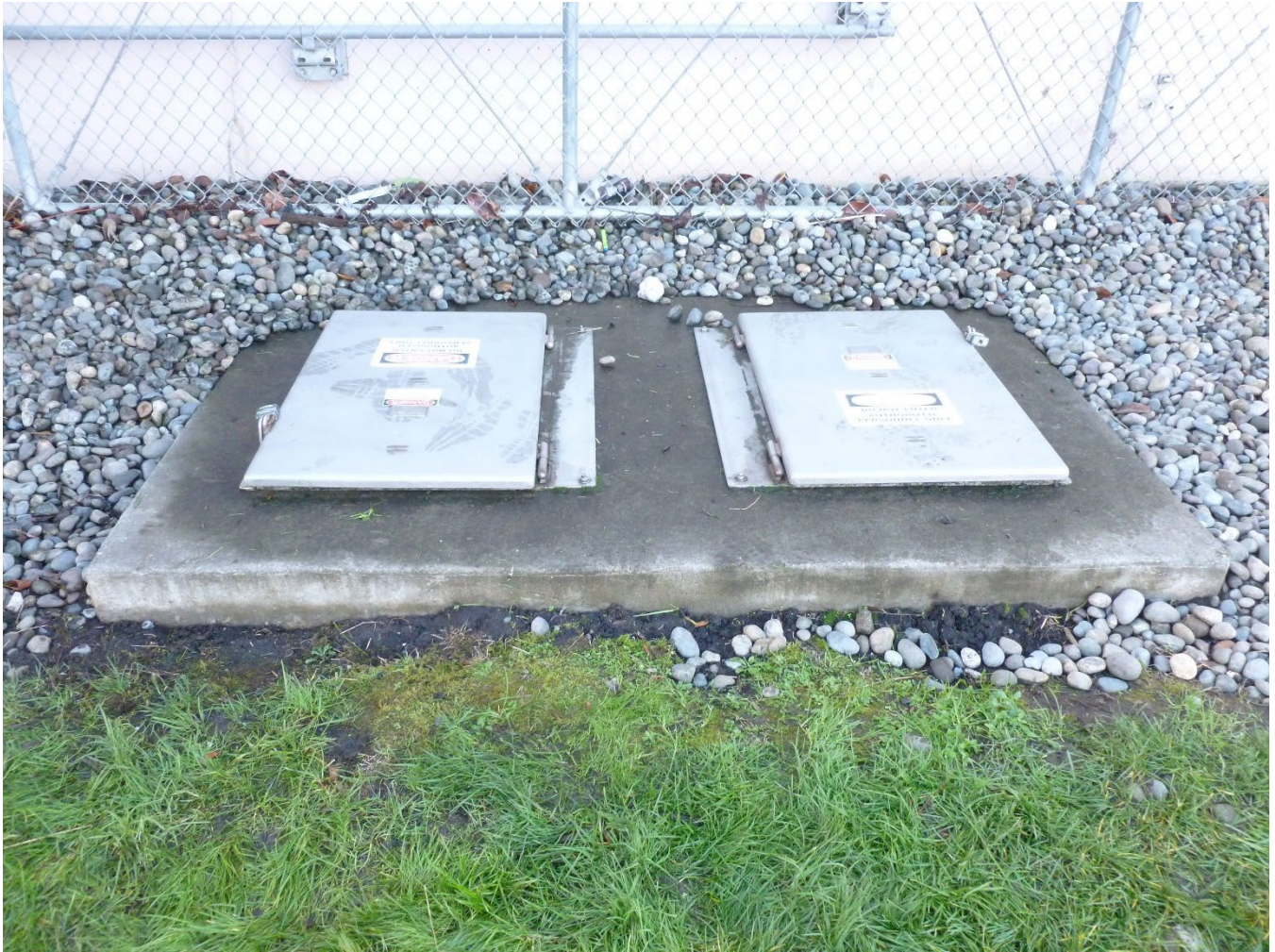
Photo 2 / P1010154 – Catch Basin 5 Vault, exterior
