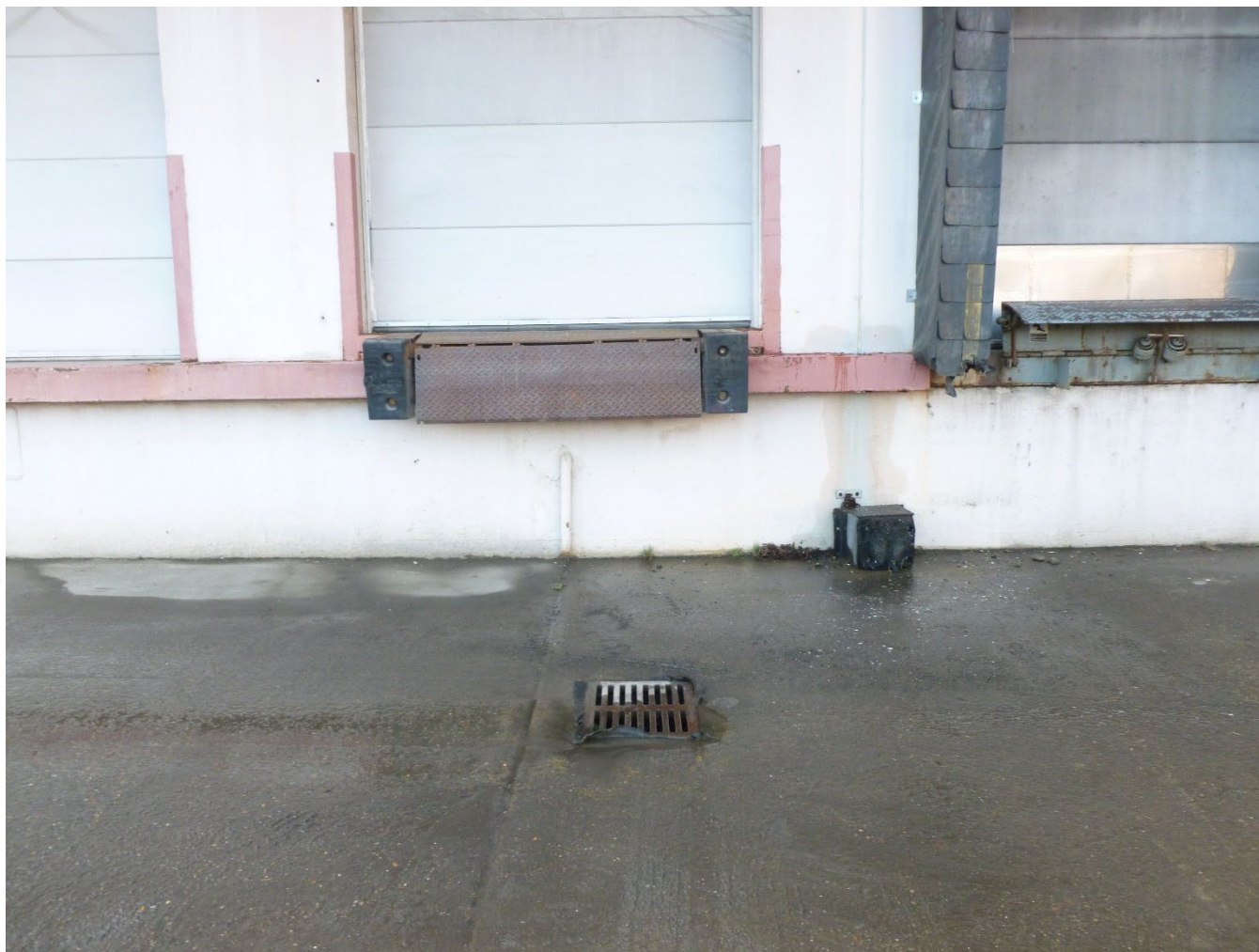
Photo 1 / P1010151 – Catch Basin 1
