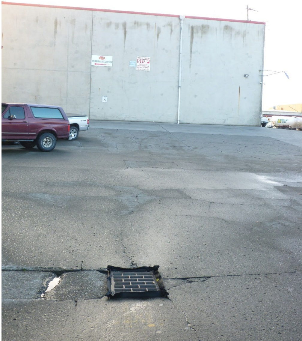
Photo 8 / P1010158 – Catch Basin 6, facing west
