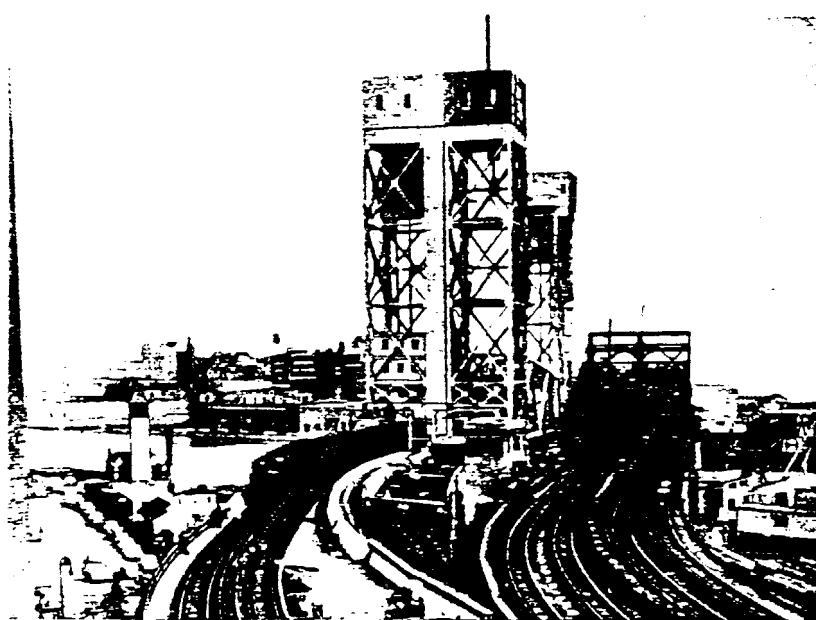
Soon to replace altogether the older bridge at right is the New York Central Railroad's twin-span lift bridge over the Harlem River in New York City. Like its predecessor, the new bridge depends upon red lead for first line protection against corrosion.
