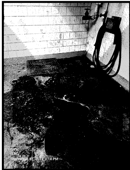
Photograph 32. Additional area of standing water on the ground in the pump room.
