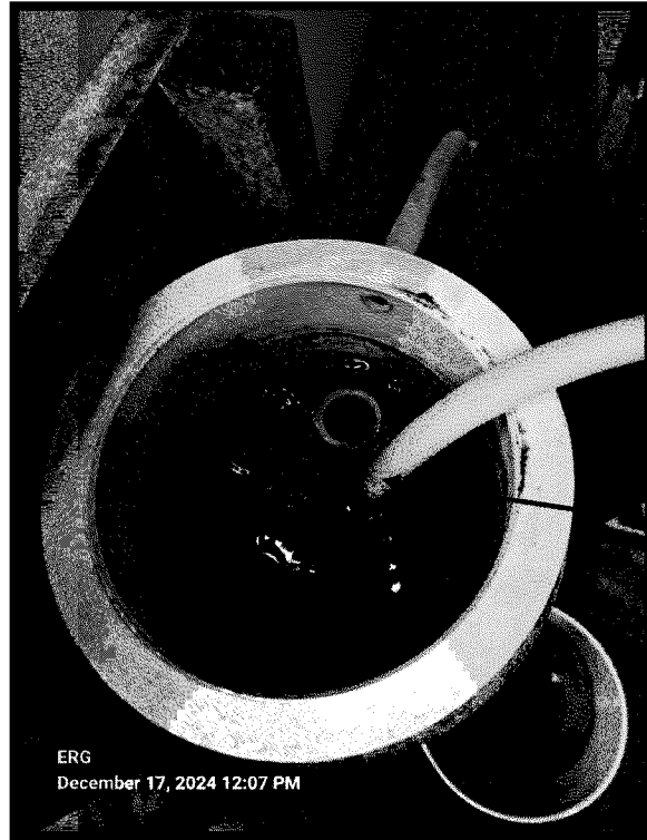
Photograph 19. Effluent sample chamber. Note the solids accumulated on the interior walls. The red arrow indicates the intake tube for the effluent auto sampler.
