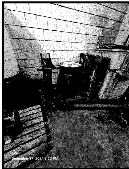
Photograph 30. Barrels filled with lubricant stored without containment. Note the brown staining down the side of the white bag on the pallet and the staining on the floor.
