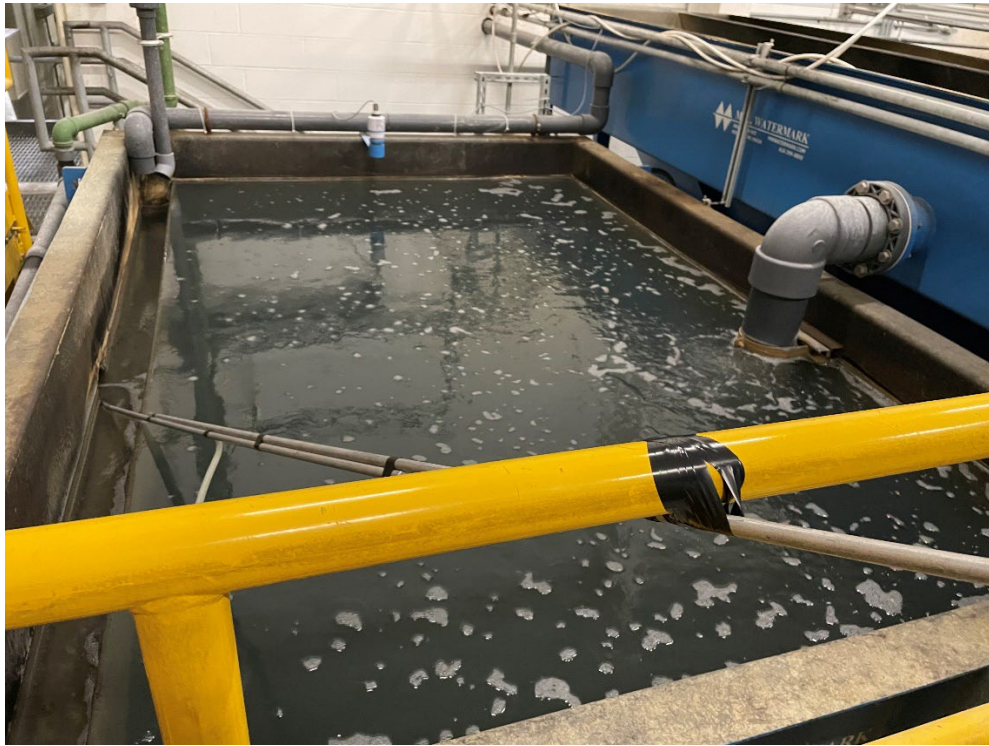
Photo #1. A 24-hr composite sample was collected of the pretreated discharged effluent.
