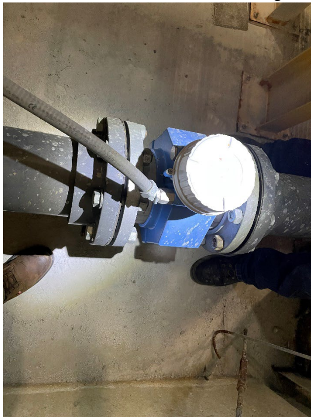
Photo #2. The magmeter monitors the effluent flow before reaching the sewer collection system.
