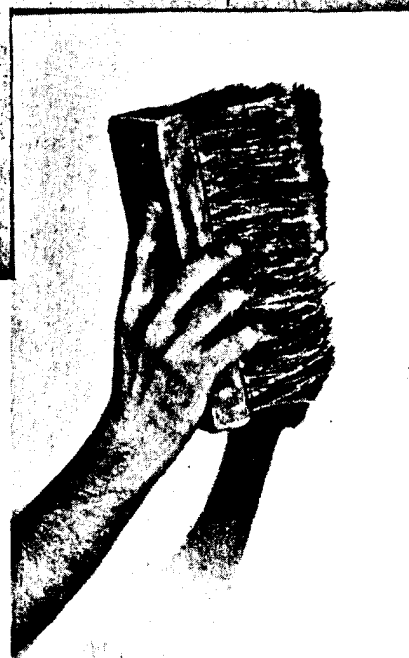
The bristle ends should all make contact with the wall surface at the same instant—brush should be held sharp and rigid.
