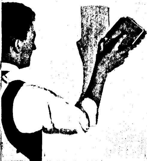
Give the brush a quarter twist of the wrist between laps. This prevents the formation of a square pattern that results when the brush is held vertically for all strokes
