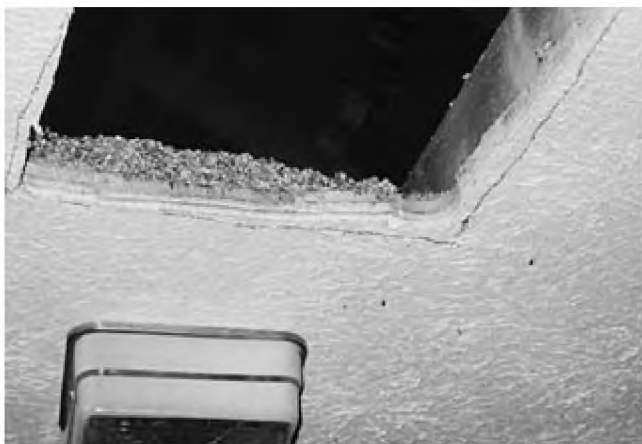
Figure 6—View of ceiling after cutting, home A.
