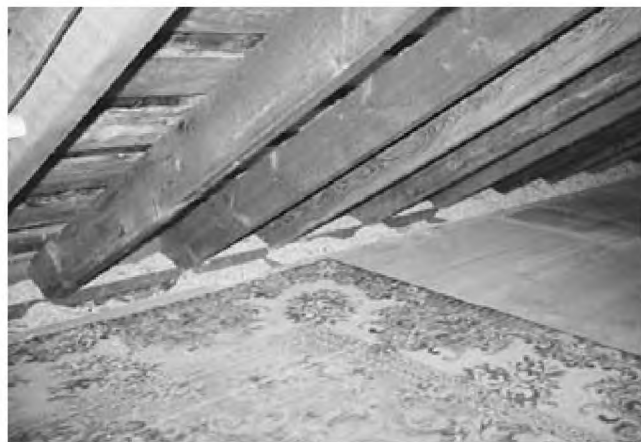
Figure 9—View of ZAI at top of wall cavity before shop vacuum removal.
