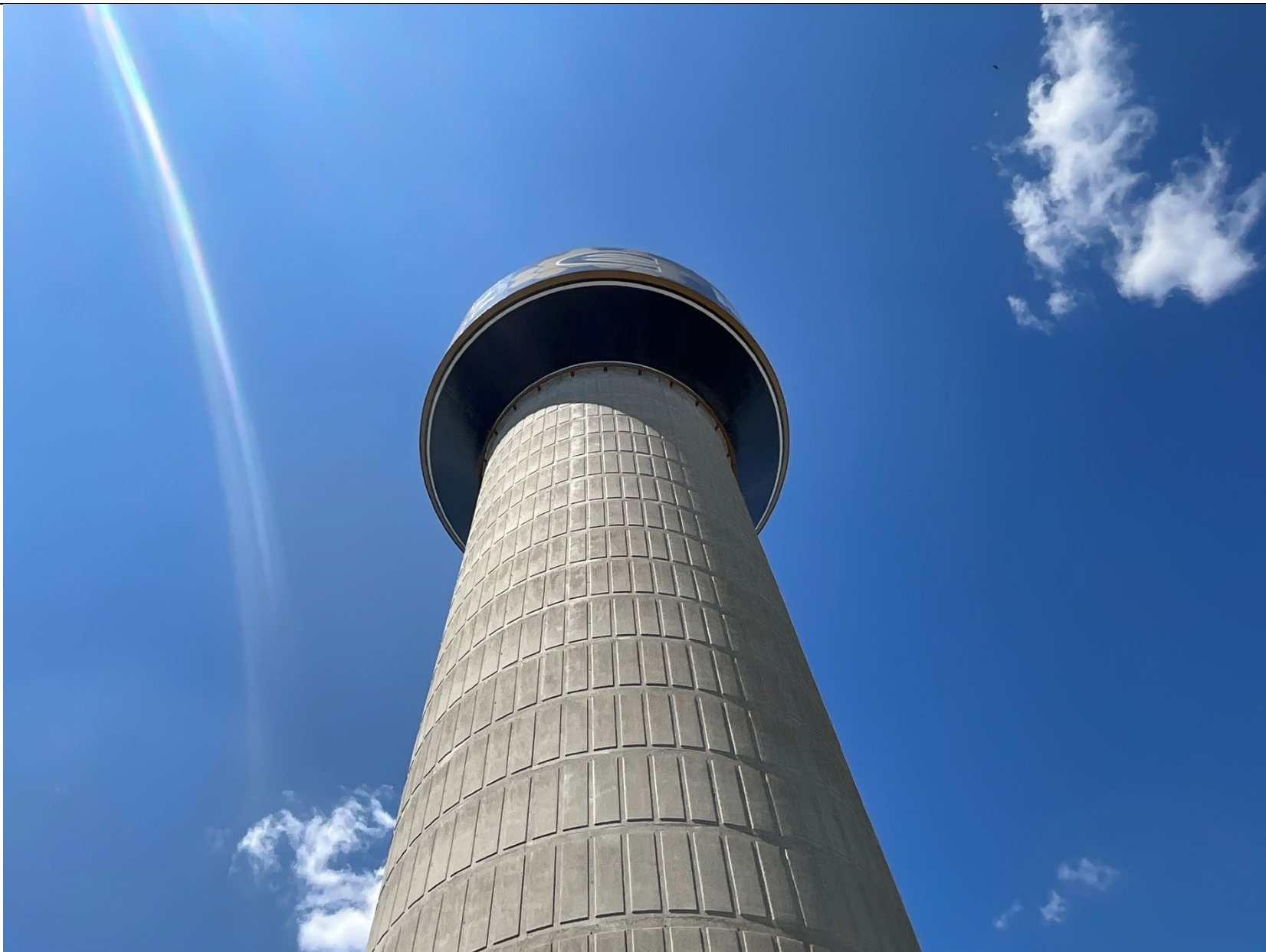
Image of the 12th Avenue elevated water storage water.
