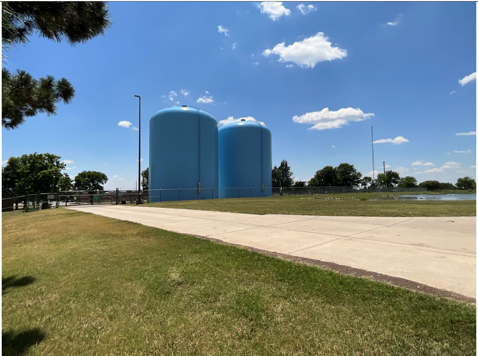
Standpipe's East and West ground storage tanks, used as clearwells prior to finished water entering the distribution system.
