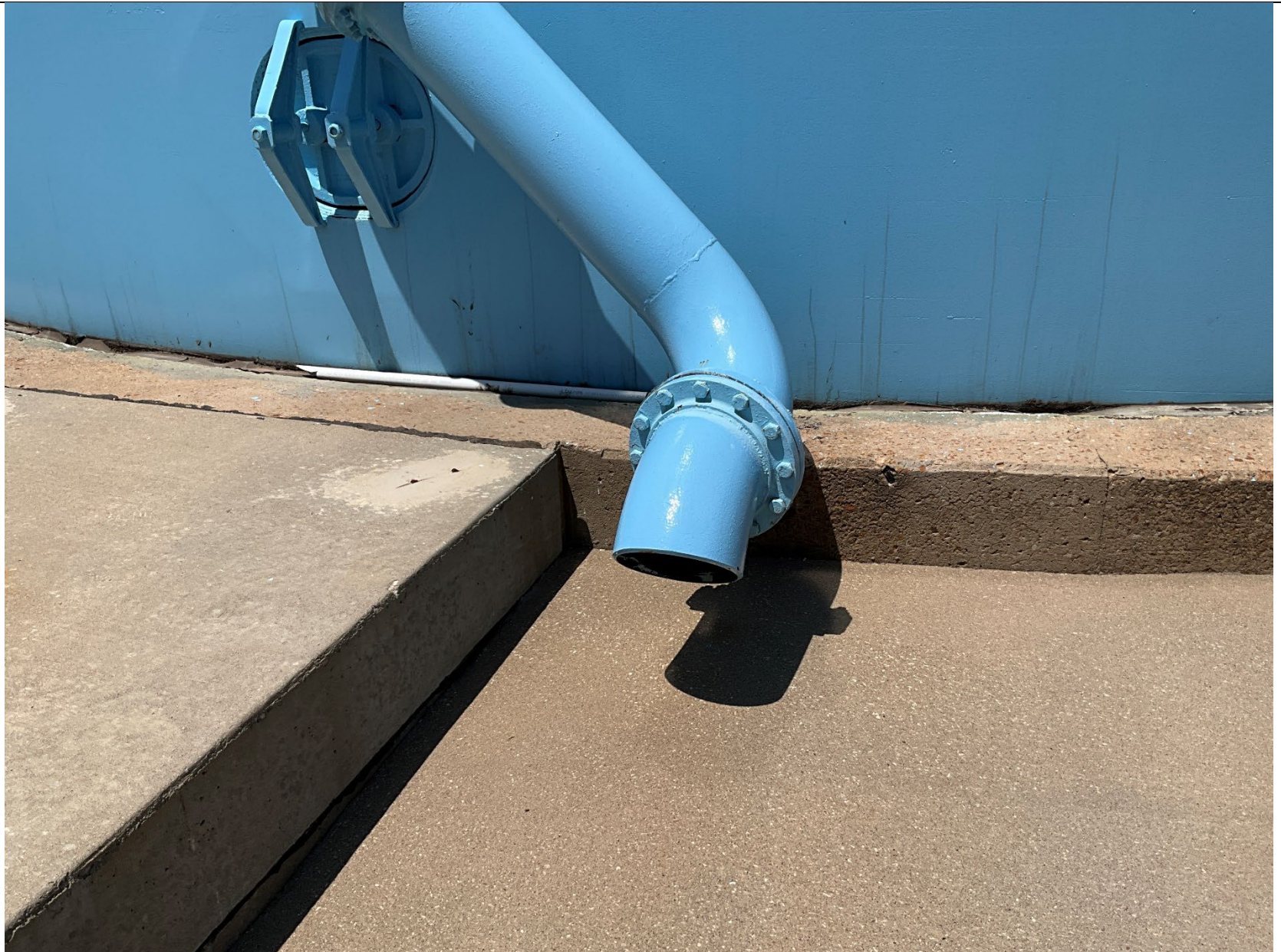
East stand pipe overflow downturned and screened.
