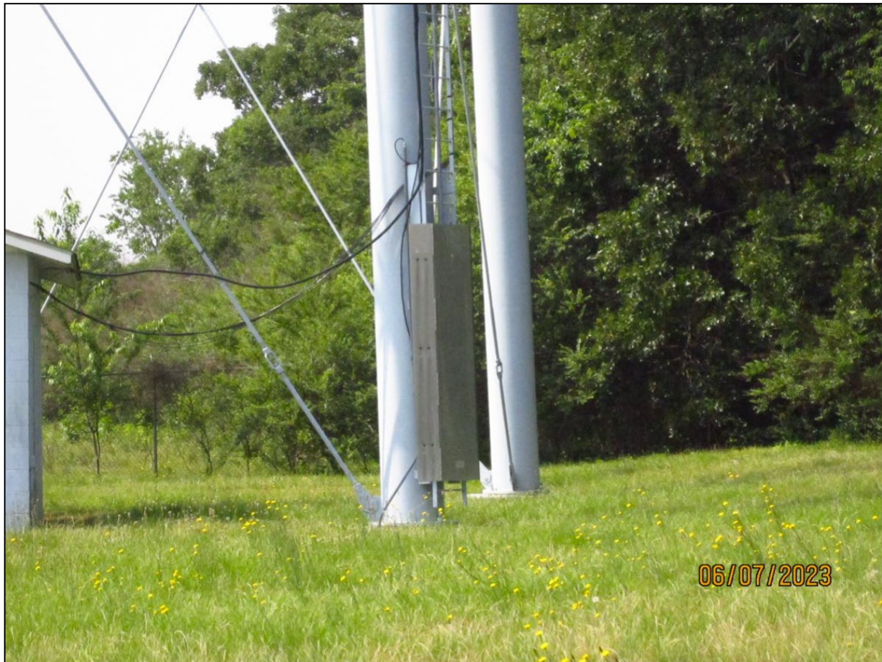
Photograph 2. Security Ladder Shield, Hopewell Water Tank View of the security shield that was covering the bottom rungs of the ladder at the Hopewell Water Tank. [REDACTED]
