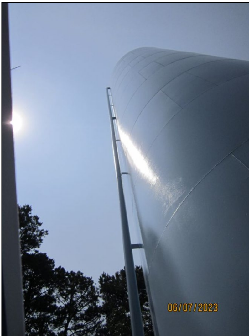
Photograph 25. Ridgecrest Water Tank View of the overflow pipe that extended off of the side of the Ridgecrest Water Tank to the ground.
