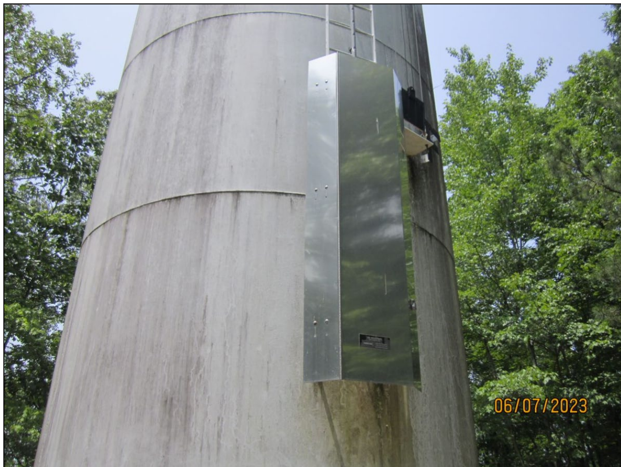
Photograph 20. Security Ladder Shield, Water Tank #1 View of the security ladder shield at Water Tank #1. The security shield was locked.
