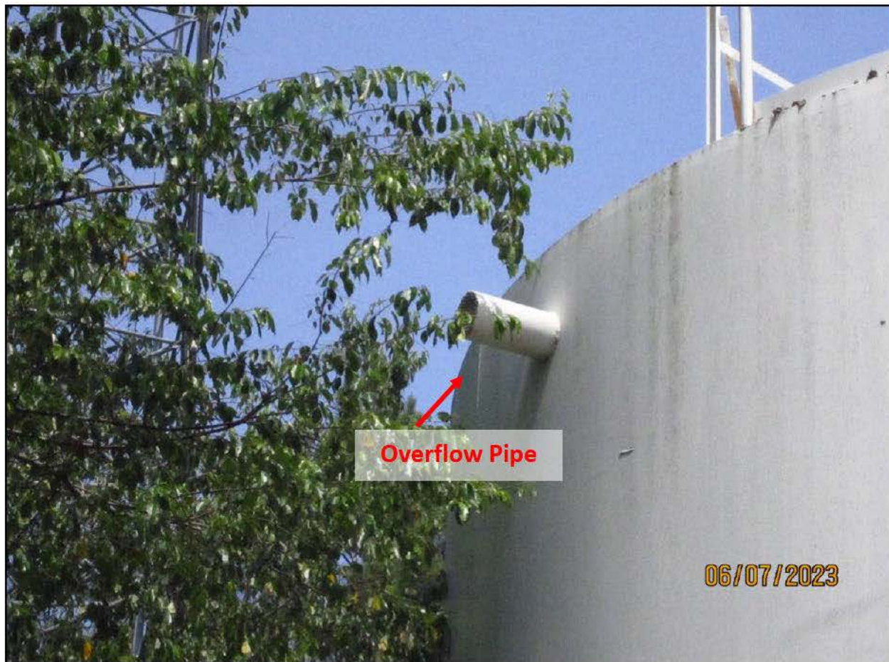
Photograph 8. Overflow Pipe, Rosebud Water Tank View of the overflow pipe that extended out of the top of the Rosebud Water Tank. There appeared to be a coarse screen over the opening of the pipe, but it was unclear what size the screen was. There was no splash pad beneath the pipe.
