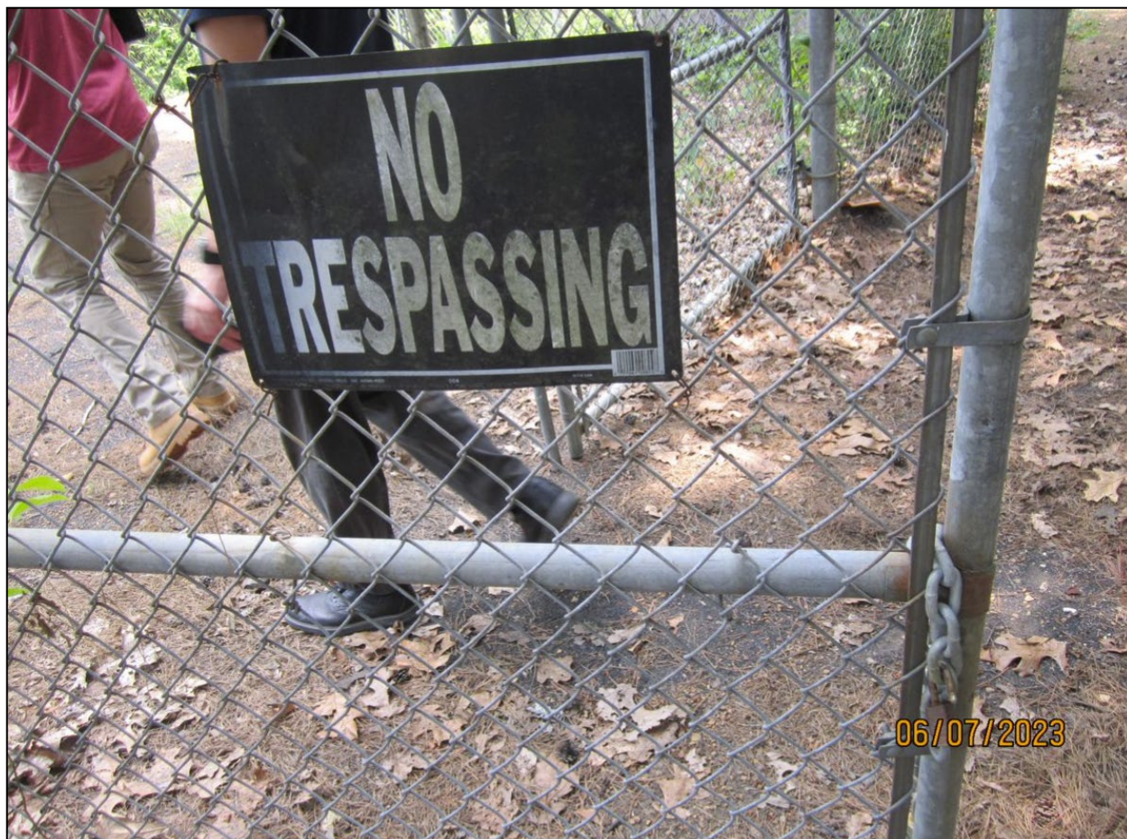
Photograph 24. Perimeter Security Fence, Ridgecrest Water Tank View of a “No Trespassing” sign that was posted on the security fence of the Ridgecrest Water Tank.
