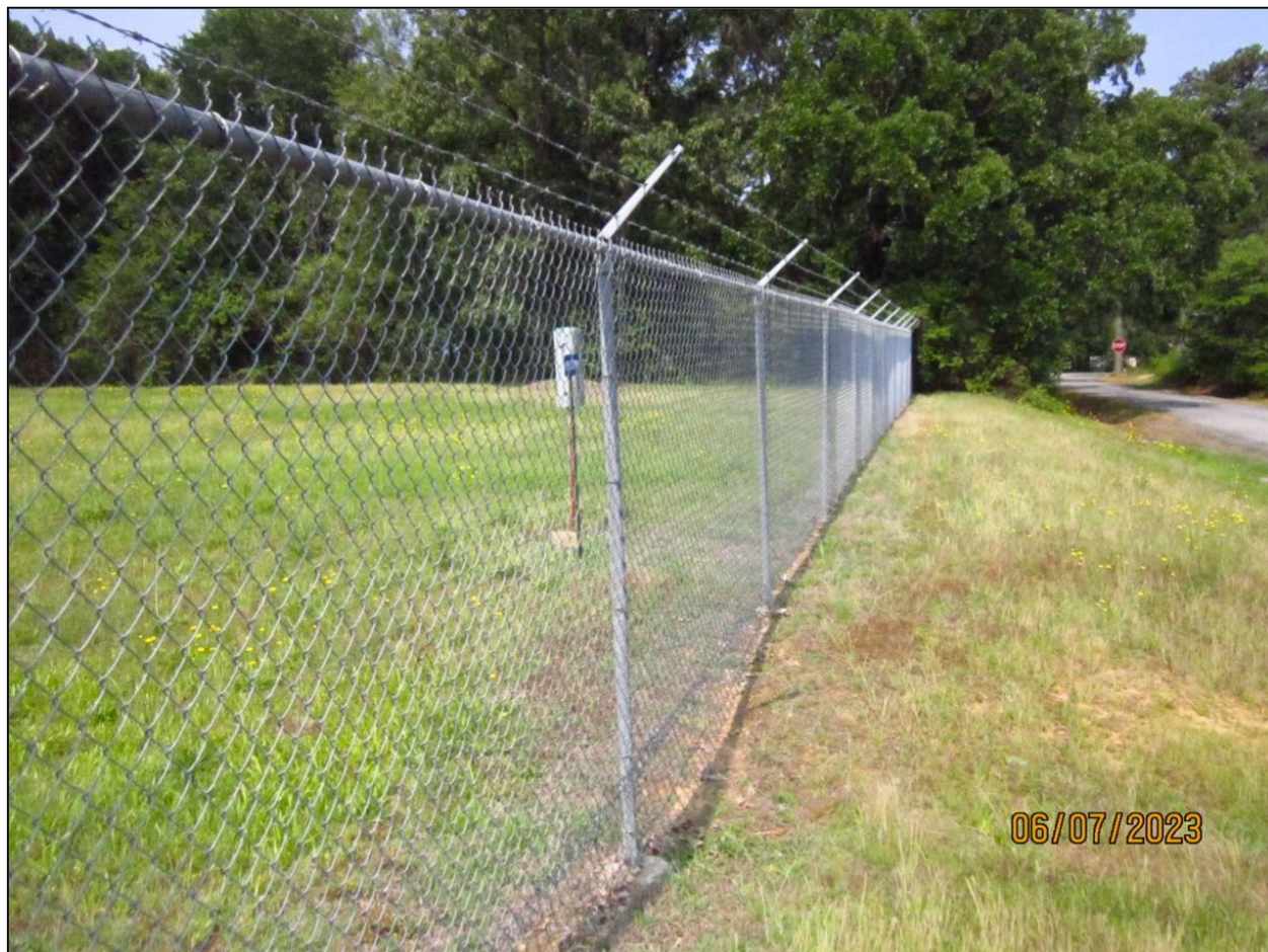
Photograph 1. Perimeter Fence, Hopewell Water Tank View of the locked perimeter fence with barbed wire that surrounded the Hopewell Water Tank. The tank was approximately 50 yards from a church.
