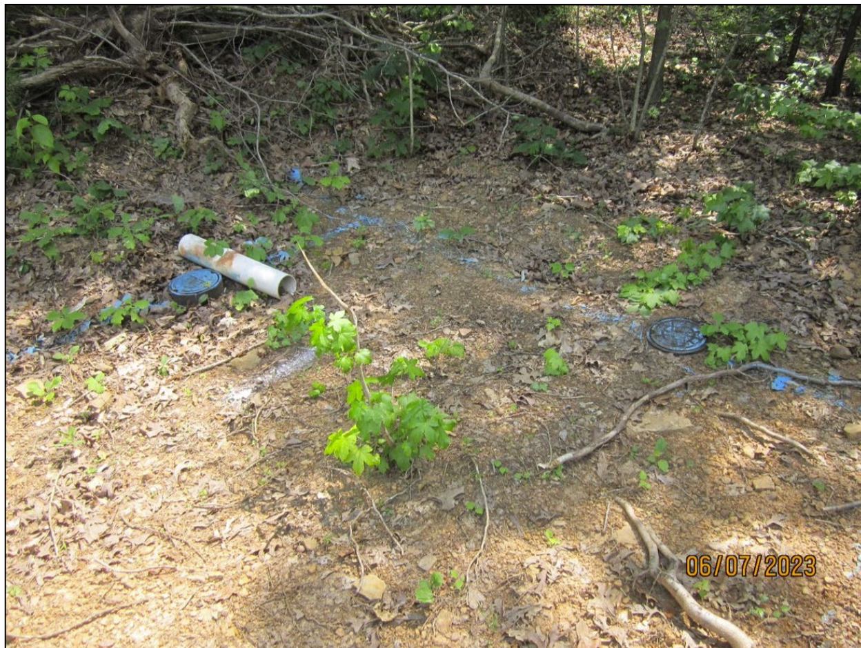
Photograph 36. Valves, Pump Station #2 View of the ground at Pump Station #2, downhill of the leaking valve. Paint showed where water lines were located so that the scheduled excavation and repairs could take place.
