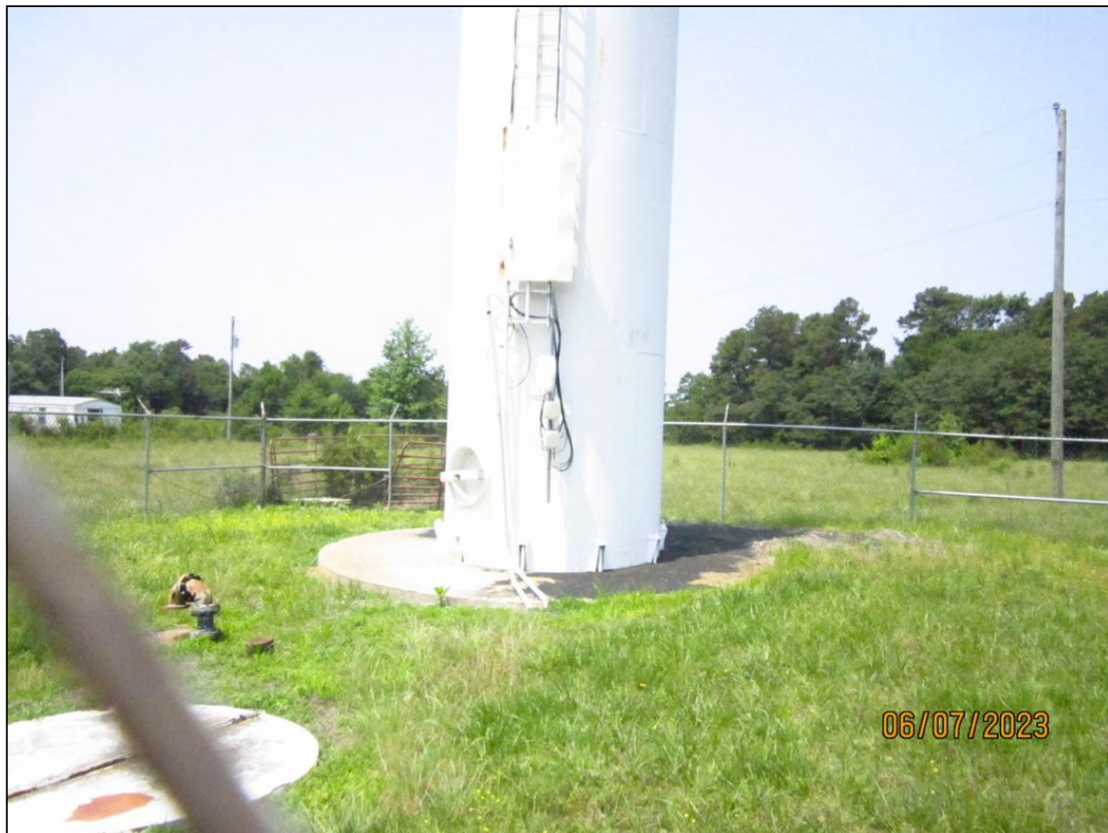
Photograph 15. Joy Water Tank View of the Joy Water Tank. The Joy Water Tank is a 28,950 gallon standpipe tank, and it was surrounded by a locked perimeter fence with barbed wire. The tank is approximately 50 yards from the nearest home.
