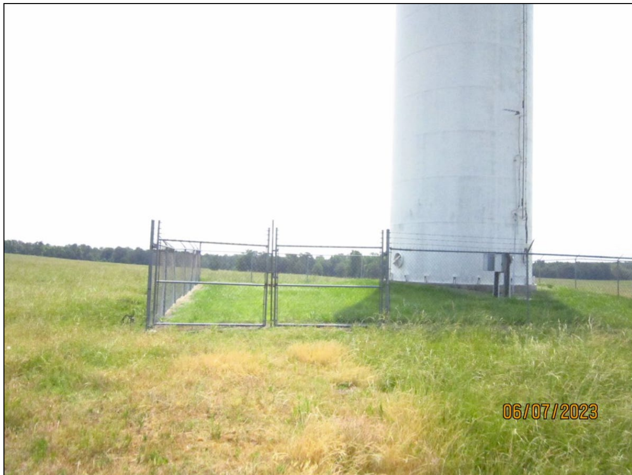
Photograph 11. Liberty Hill Water Tank View of the Liberty Hill Water Tank located in an open field approximately 150 yards from local homes. The Liberty Hill Water Tank is a 199,400 gallon standpipe tank, and it was surrounded by a locked perimeter fence with barbed wire.
