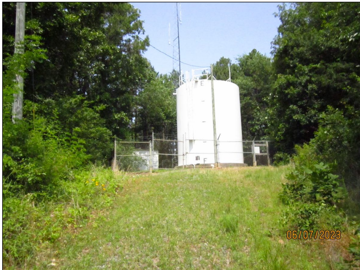
Photograph 5. Rosebud Water Tank View of the Rosebud Water Tank located at the end of a grass covered dirt and graveled road in a heavily wooded, undeveloped area. The tank is 59,000 gallons and was surrounded by a locked perimeter fence.
