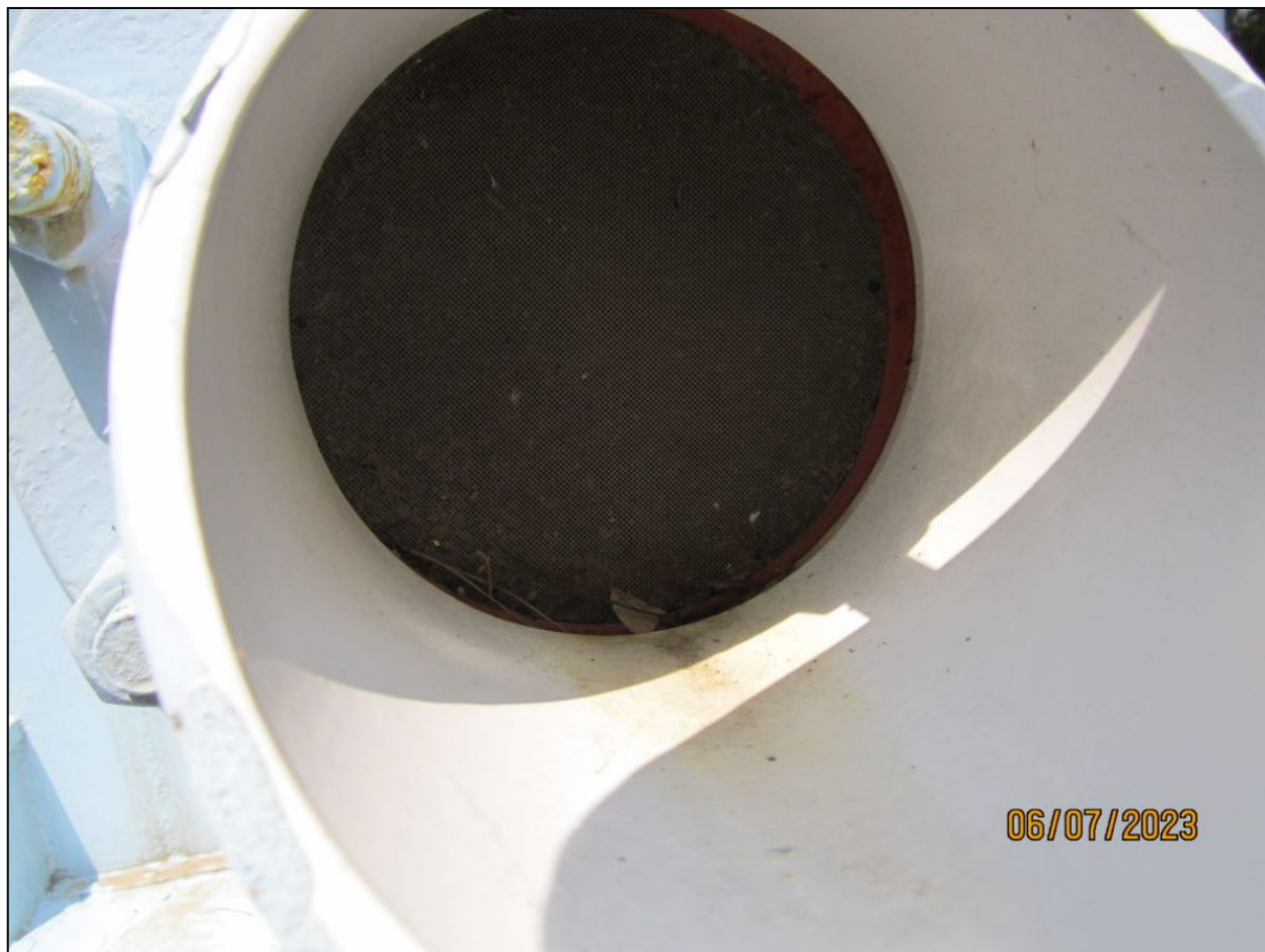
Photograph 27. Overflow Pipe, Ridgecrest Water Tank View of the inside of the overflow pipe that extended off of the Ridgecrest Water Tank. The opening was covered by a 24-inch mesh screen beneath a flapper valve.
