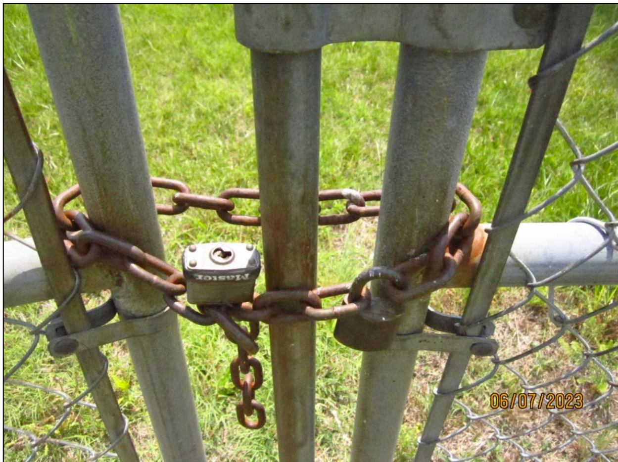
Photograph 12. Perimeter Fence Lock, Liberty Hill Water Tank View of the locks on the security fence that was surrounding the Liberty Hill Water Tank. The fence also contained barbed wire.
