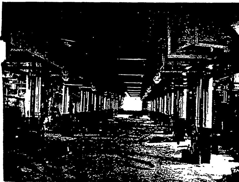
One of the first manufacturing plants when under construction at Deepwater, N. J. in 1926. This building is no longer used.
