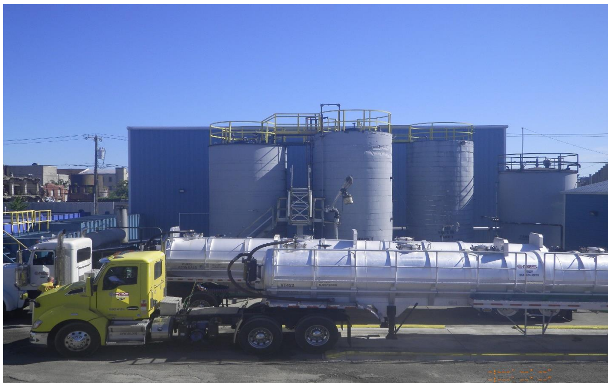
10. Truck Loading/Unloading Area and Oil Tanks – PRC – 09/14/22
