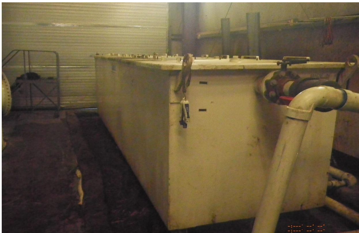
6. Oil/Water Separator for Industrial Wastewater - PRC – 09/14/22
