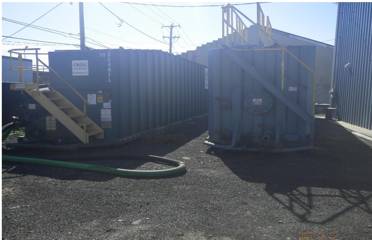
9. Portable Frac Liquid Settling Tanks – PRC – 09/14/22
