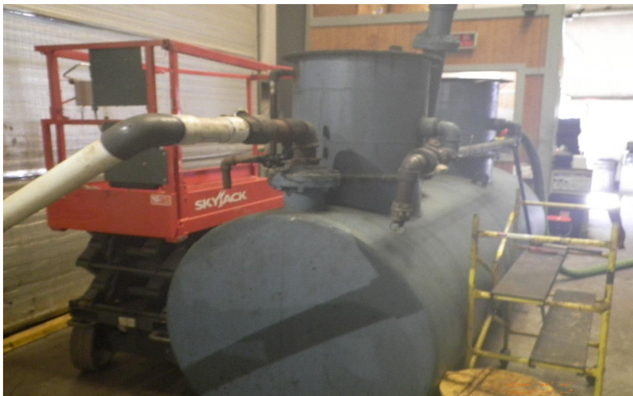
7. Oil/Water Separator for Industrial Wastewater – PRC – 09/14/22
