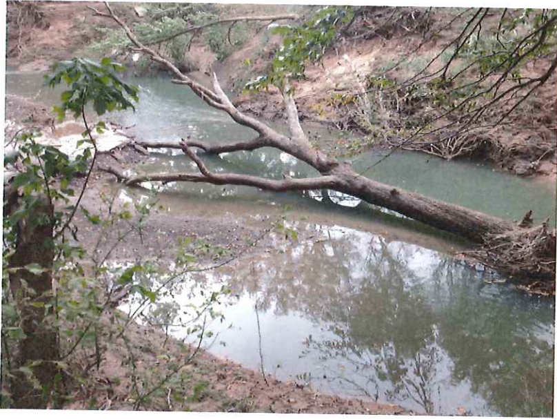
Pictures of Creek the Day we found the Break
