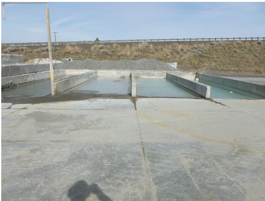
Photo 2/P1010290 – Truck Washout
