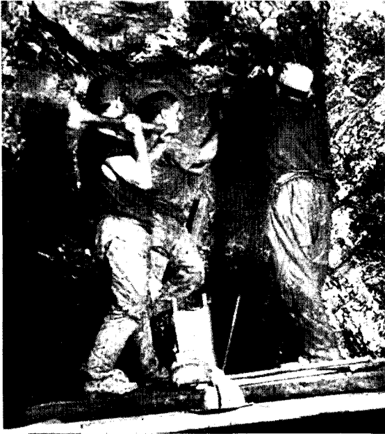
PLATE III.—Hand drilling (drifting).
