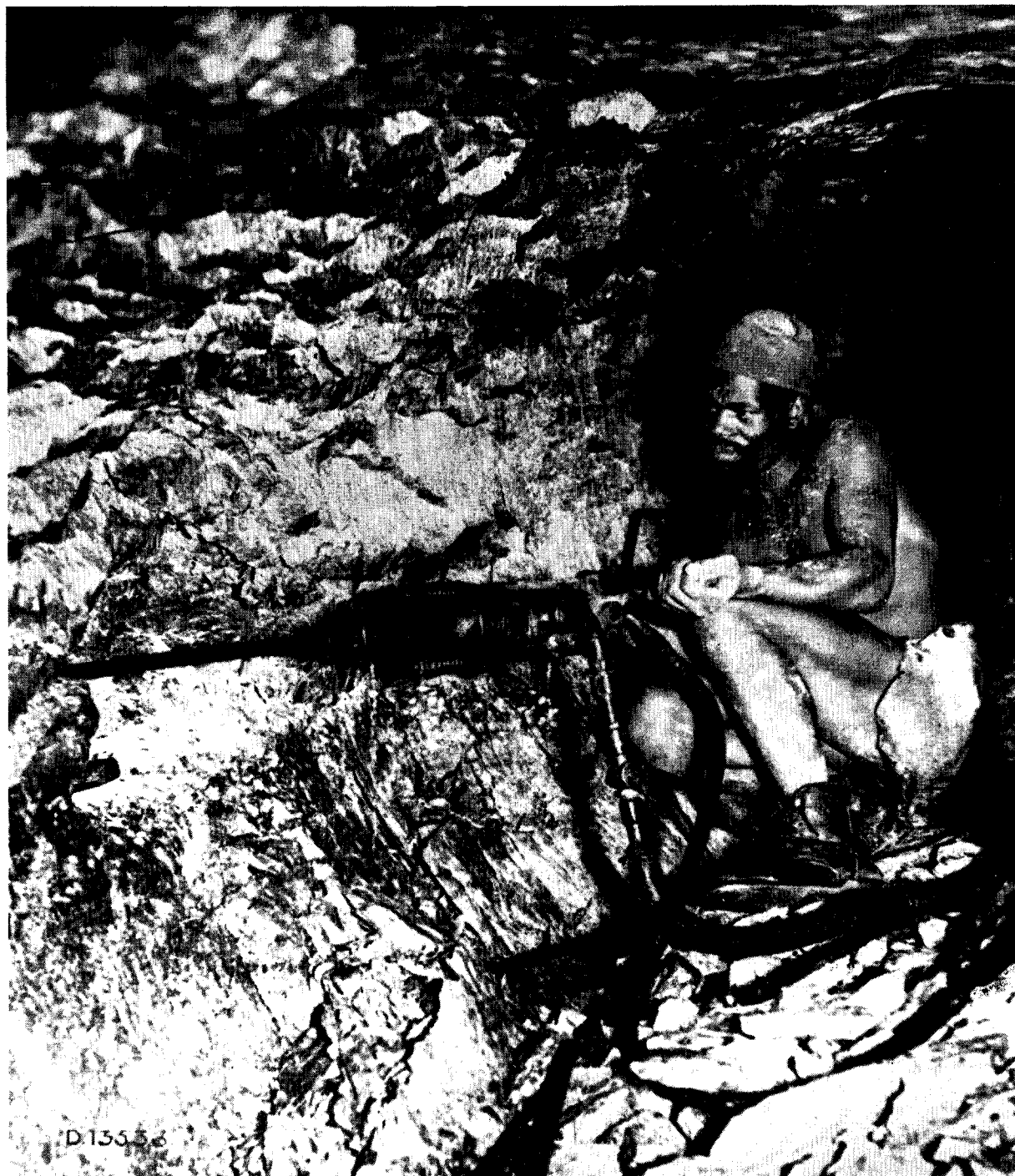
PLATE XXVII.—Underhand stoping on Witwatersrand with vented drill (note air and water hoses).
