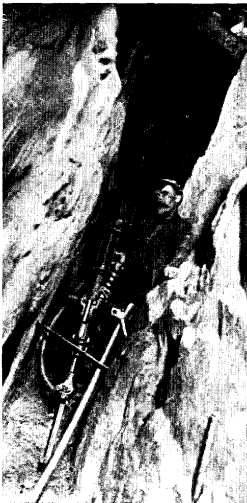
PLATE XX.—Drill of 1905 at work in narrow underhand stope (dry).
