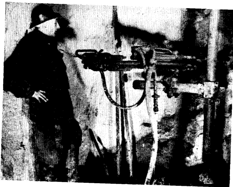
PLATE XVIII.—Automatic vented drifter drill of 1945 with single control for air and water.
