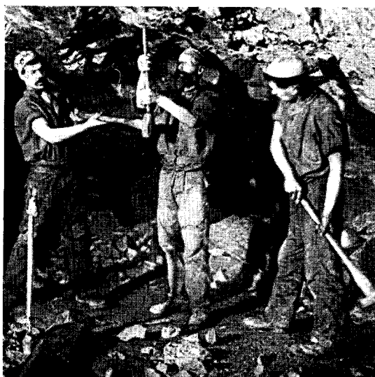
PLATE XXVIII—Hand drilling, overhand stoping.
