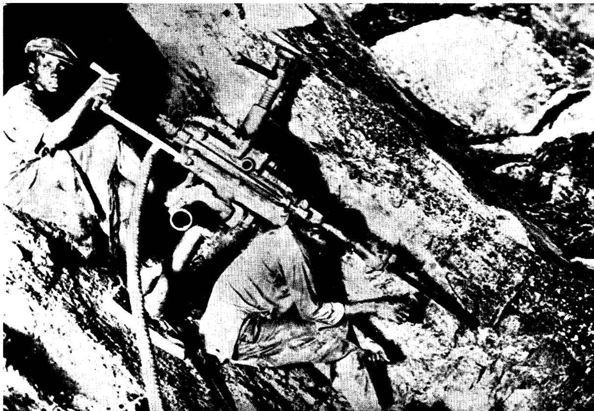
PLATE XI.—Early method of introducing water into hole.
