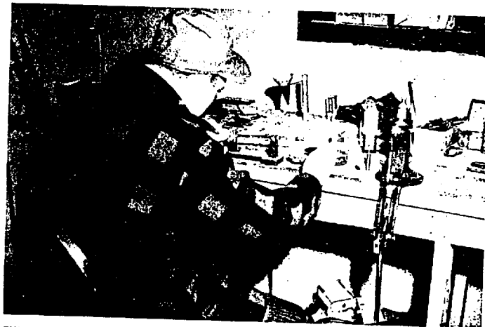
THE MOST DELICATE part of making "home-made bullets" is weighing of the gunpowder (above). Too much powder could damage a gun — injure a shooter.
