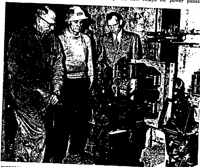
MODERN METHODS require large and expensive equipment. Above, Ashland's Norman Weis and Harry Perkins learn how to operate new type air circuit breakers.
