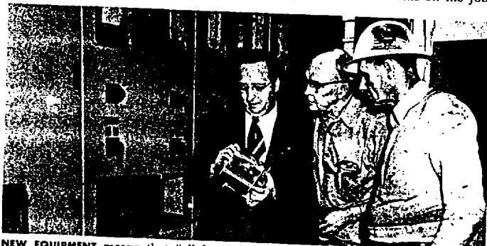
NEW EQUIPMENT means that "all hands", must be trained to operate it. Above, Guy Coffman, Ashland Power Engineer, explains new relays for power panels.
