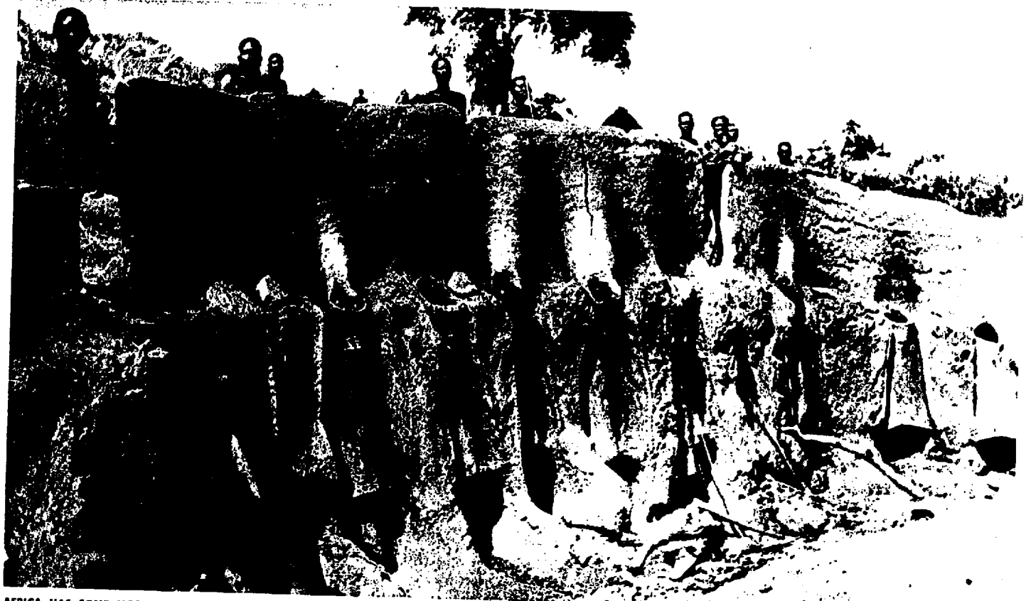
AFRICA HAS SOME MODERN, EFFICIENT BLAST FURNACES. BUT IT ALSO HAS SOME OF THESE CRUDE CLAY ONES, TOO, WHERE IRON IS STILL BEING MADE IN THE OLD WAY.
