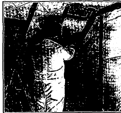
Applying J-M Home Insulation bats in new home
