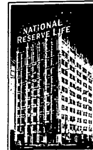
10-Story Office Building at Topeka, Kan., Air Conditioned Throughout with Frick Freon Refrigeration
