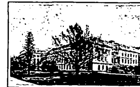
Four Frick Freon Compressors, Totalling 780 Tons Refrigeration, are used in Air Conditioning the Wings of the Administration Building of the Department of Agriculture, at Washington, D. C.
