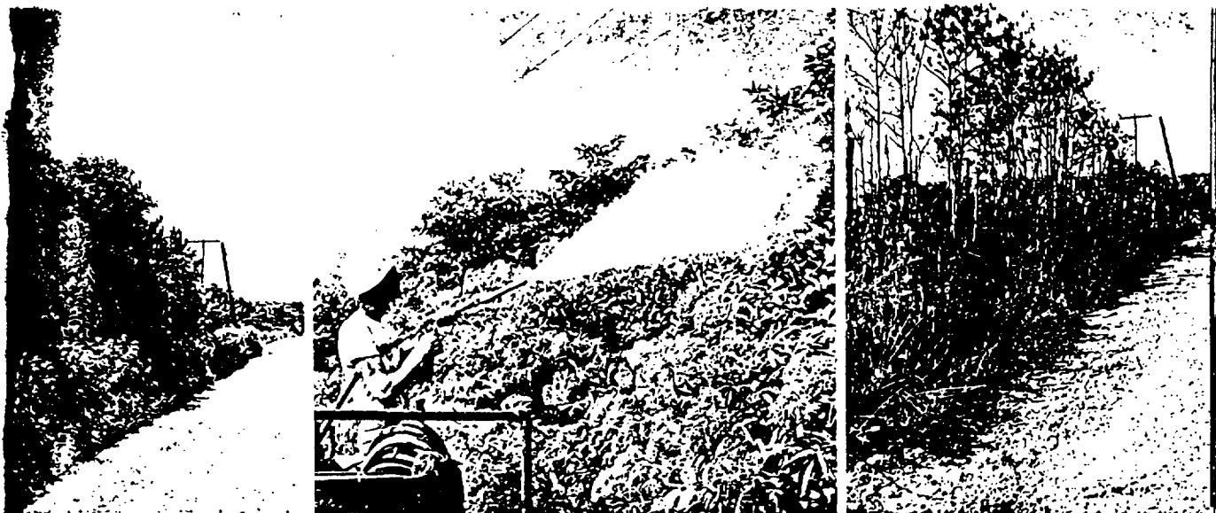
How utility rights-of-way are cleared of brush by TORDON herbicide spraying is shown in these before and after photos.
