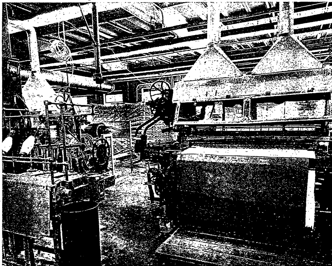
Fig. 3.—Automatic cloth loom, showing exhaust hood.
