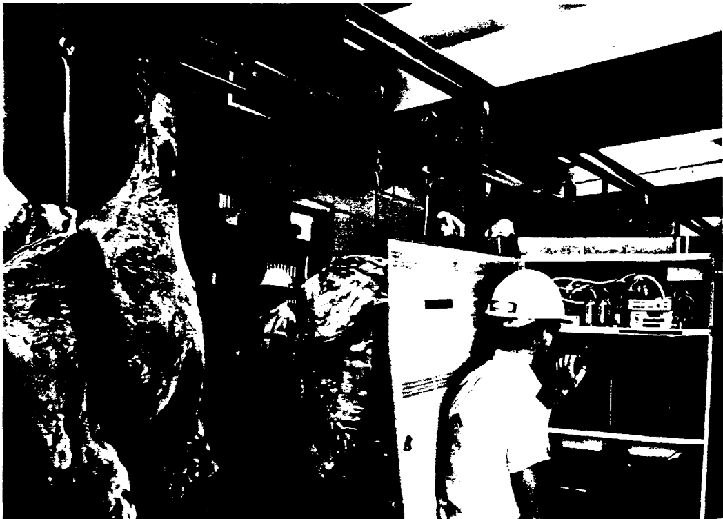
Technician seen in left view checks centrally located console system used to power emergency fluorescent lighting in meat processing plant. Insert view shows close-up of battery-powered system.
