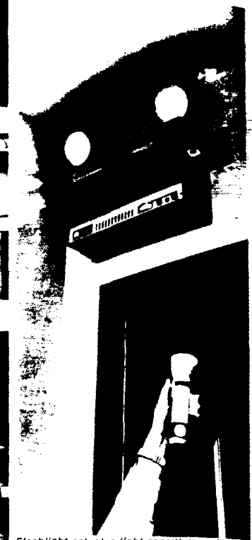
Flashlight actuates light-sensitive mechanism used to test battery powered emergency lighting system.
