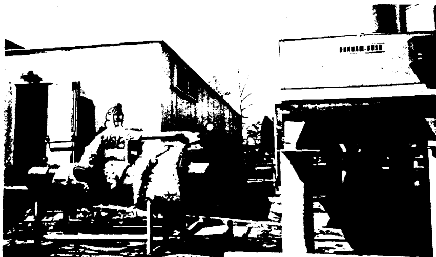
Regulating station undergoes testing at Jerome UTE. Heat exchanger equipment is at right.
