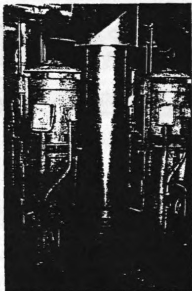
Right out in the open are three Elliott 1500-hp, 3600-rpm weather-protected induction motors driving the boiler-feed pumps. A portion of the Unit 3 turbine-generator unit is seen at top left.
