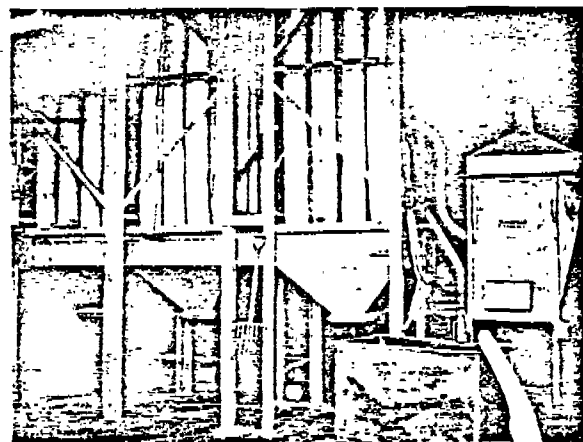
Scrap cutter hood and dust collector.
