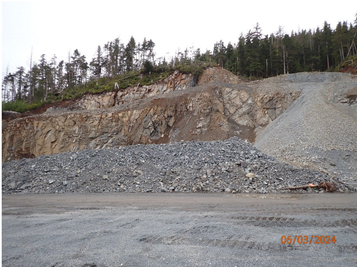
Photo 1 - Drilling and blasting area
