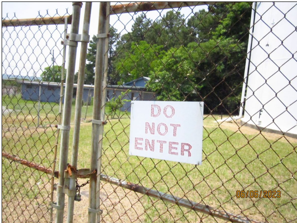
Photograph 3. North Water Tank Perimeter Fence View of a "Do Not Enter" sign that was posted on the locked perimeter fence of the North Water Tank.
