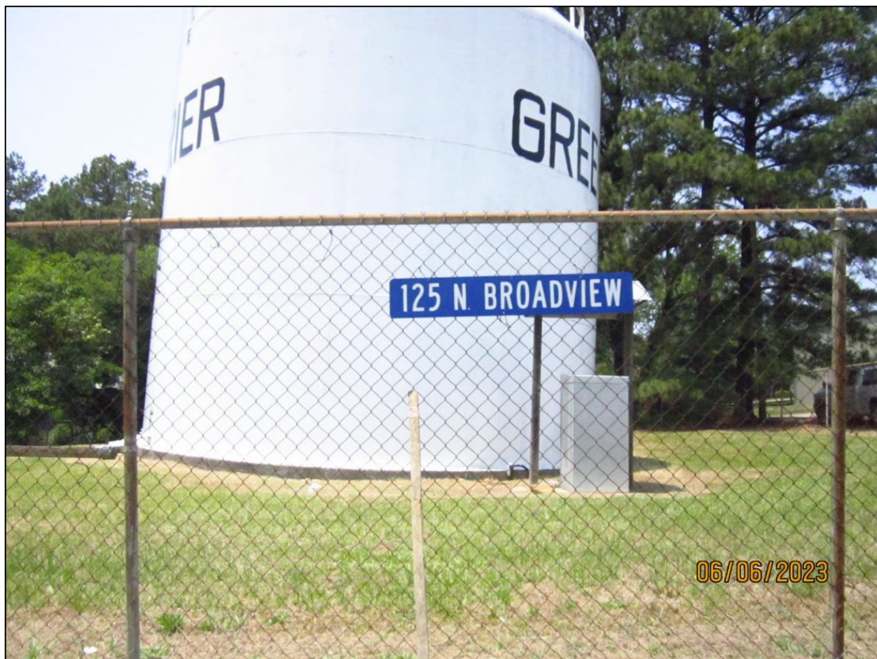
Photograph 1. North Water Tank View of the North Water Tank. The tank is 100,000 gallons and was surrounded by a locked perimeter fence.
