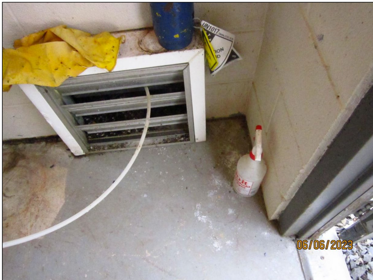
Photograph 24. Chlorinator Vent Line, Master Meter #2 View of a chlorinator vent line in the chlorine storage room at Master Meter #2. The chlorinator vent lines were run through the exhaust vent moveable louvers. It was unclear if the lines would negatively impact the room's designed ability to properly manage a release of chlorine gas.
