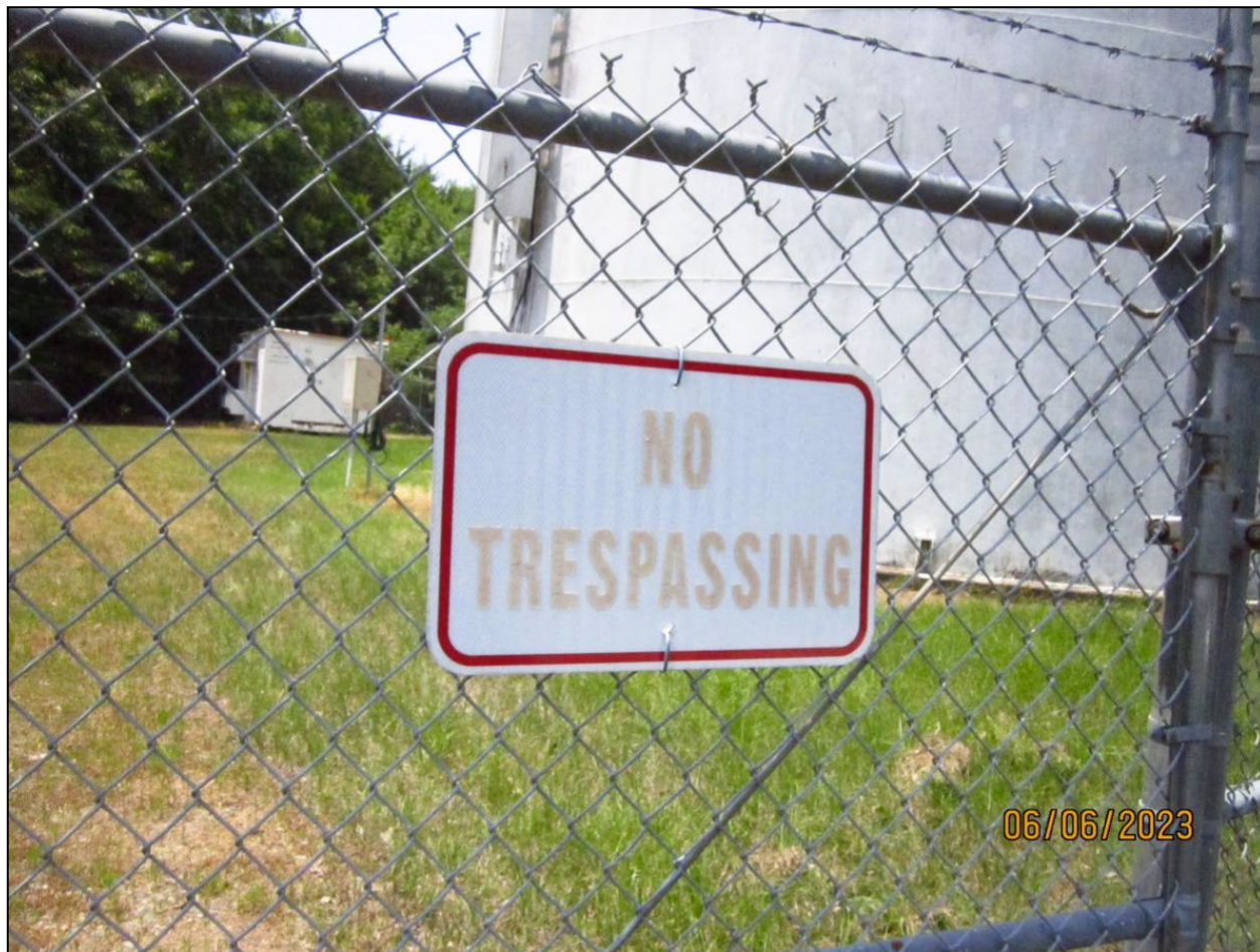
Photograph 7. Horseshoe Mountain Tank Perimeter Fence View of a "No Trespassing" sign that was posted on the locked perimeter fence of the Horseshoe Mountain Water Tank.
