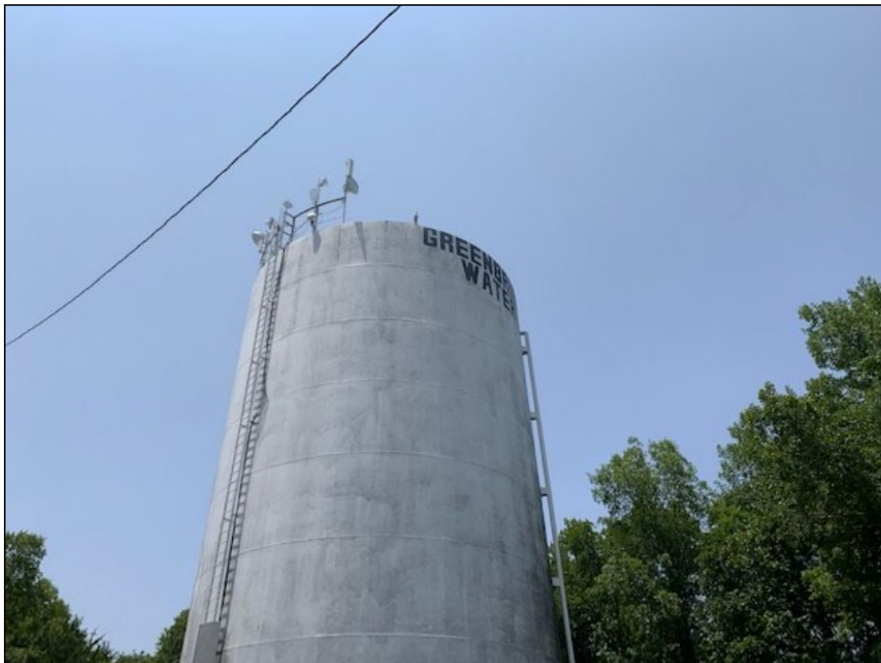
Photograph 6. Horseshoe Mountain Water Tank View of the Horseshoe Mountain Water Tank. The tank is 100,000 gallons and was surrounded by a locked perimeter fence.
