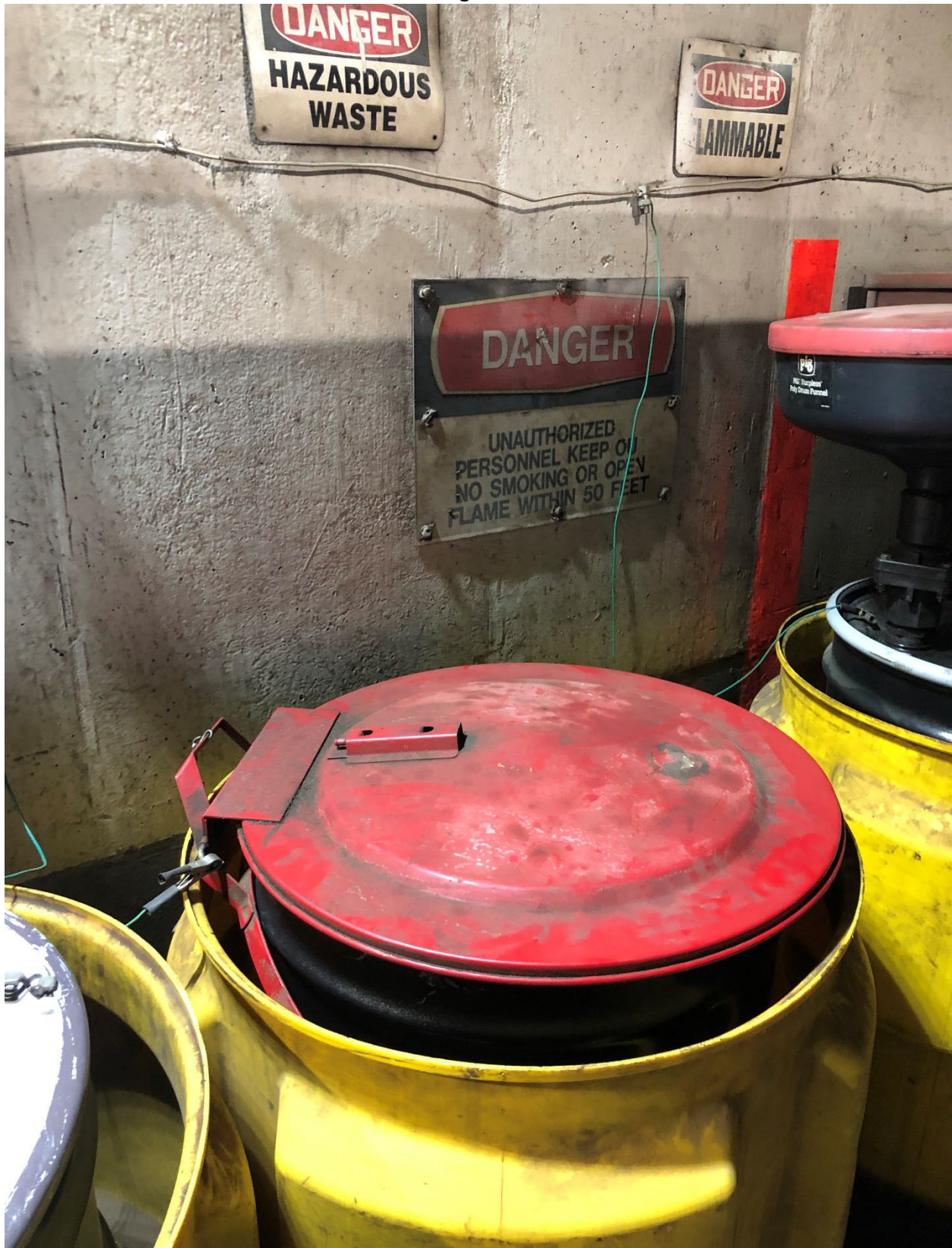
Photo #1: View of the hazardous waste storage area.
