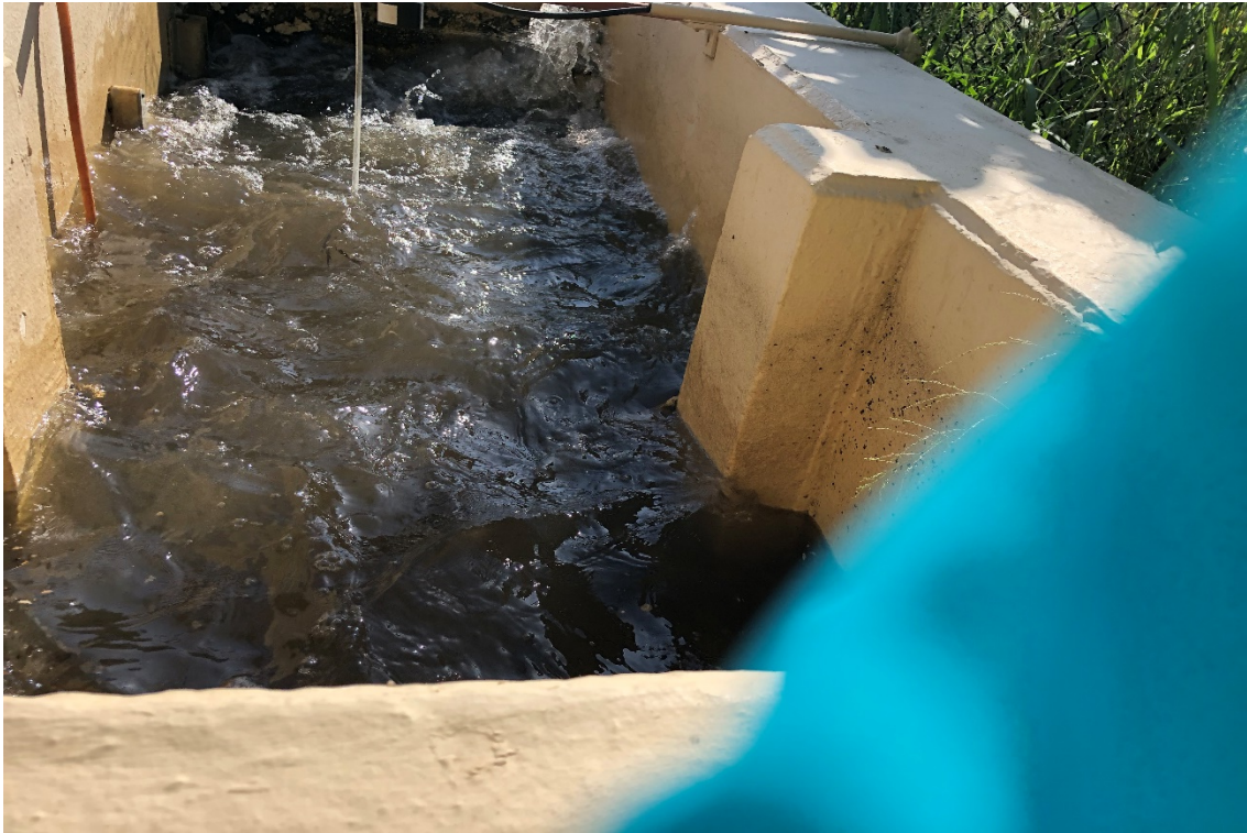
Photo #11. Flow is not recorded because the flow monitoring equipment are not operating.
