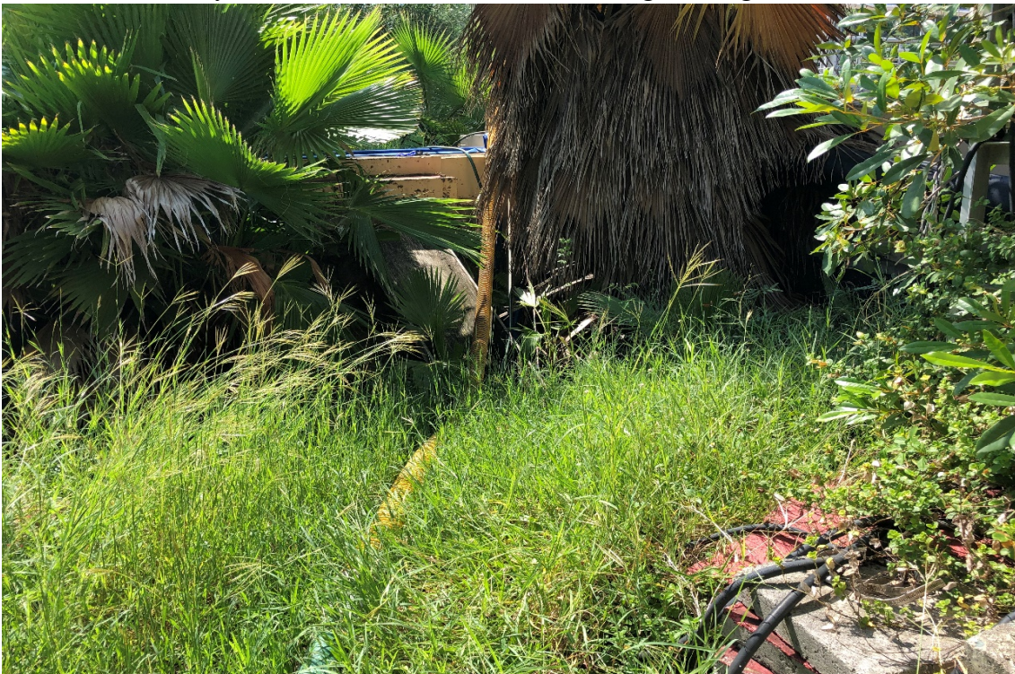
Photo #4. The walkway to the bar screen is covered with vegetative growth.
