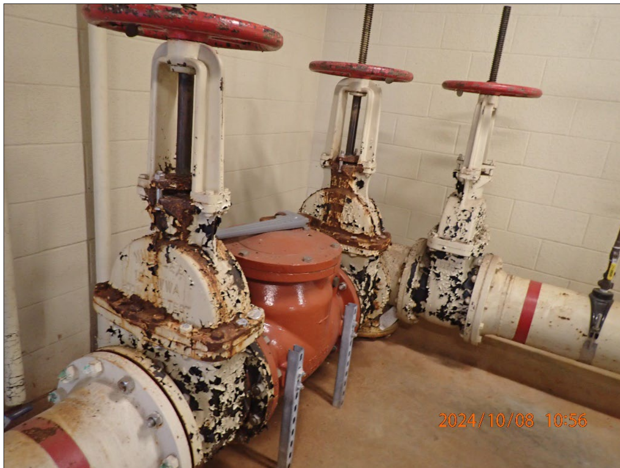
Photograph 3. West Gate Elevated Storage Tower 10/08/2024 10:56 PA080201.JPG
