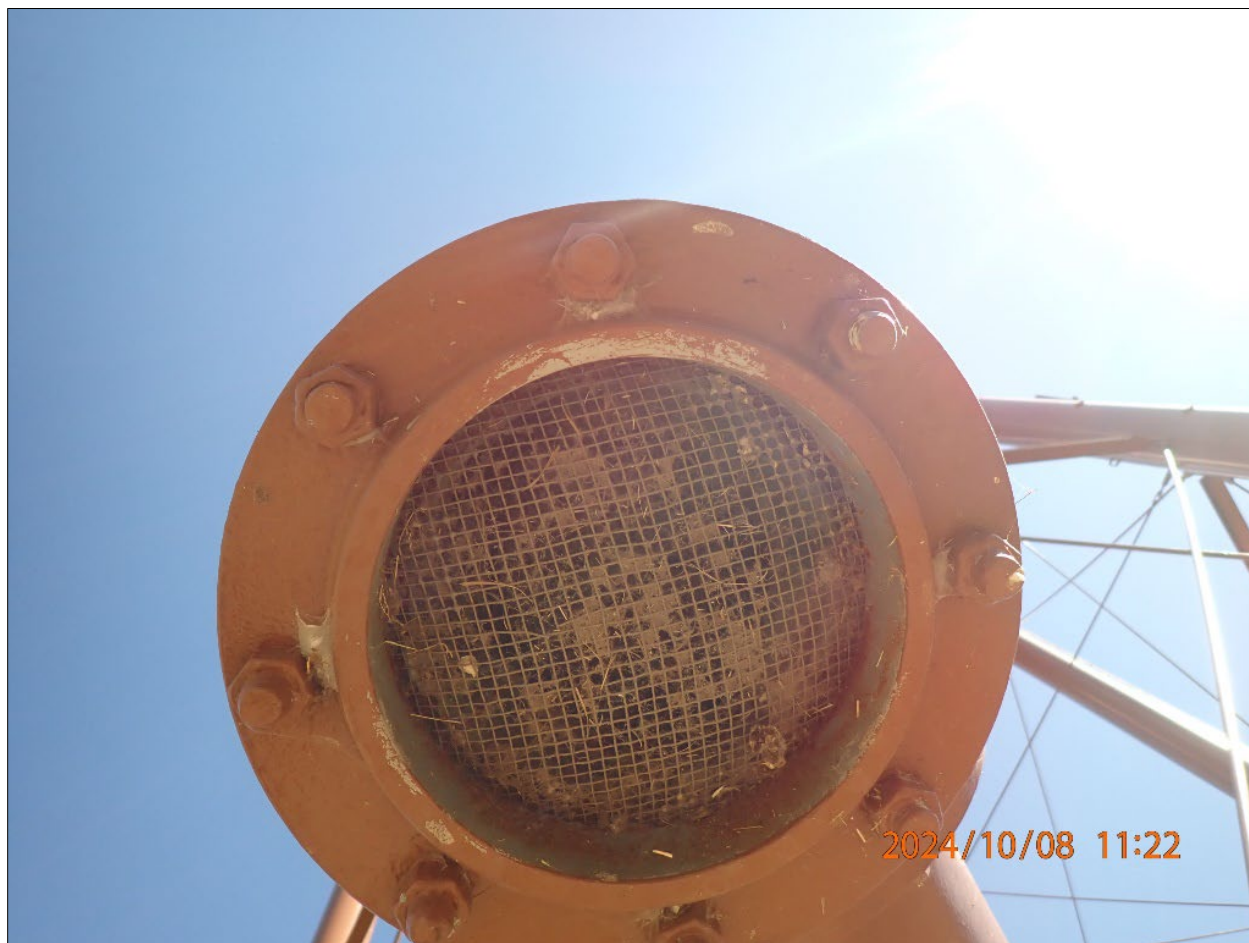
Photograph 4. Supply Elevated Storage Tower 10/08/2024 11:22 PA080215.JPG
