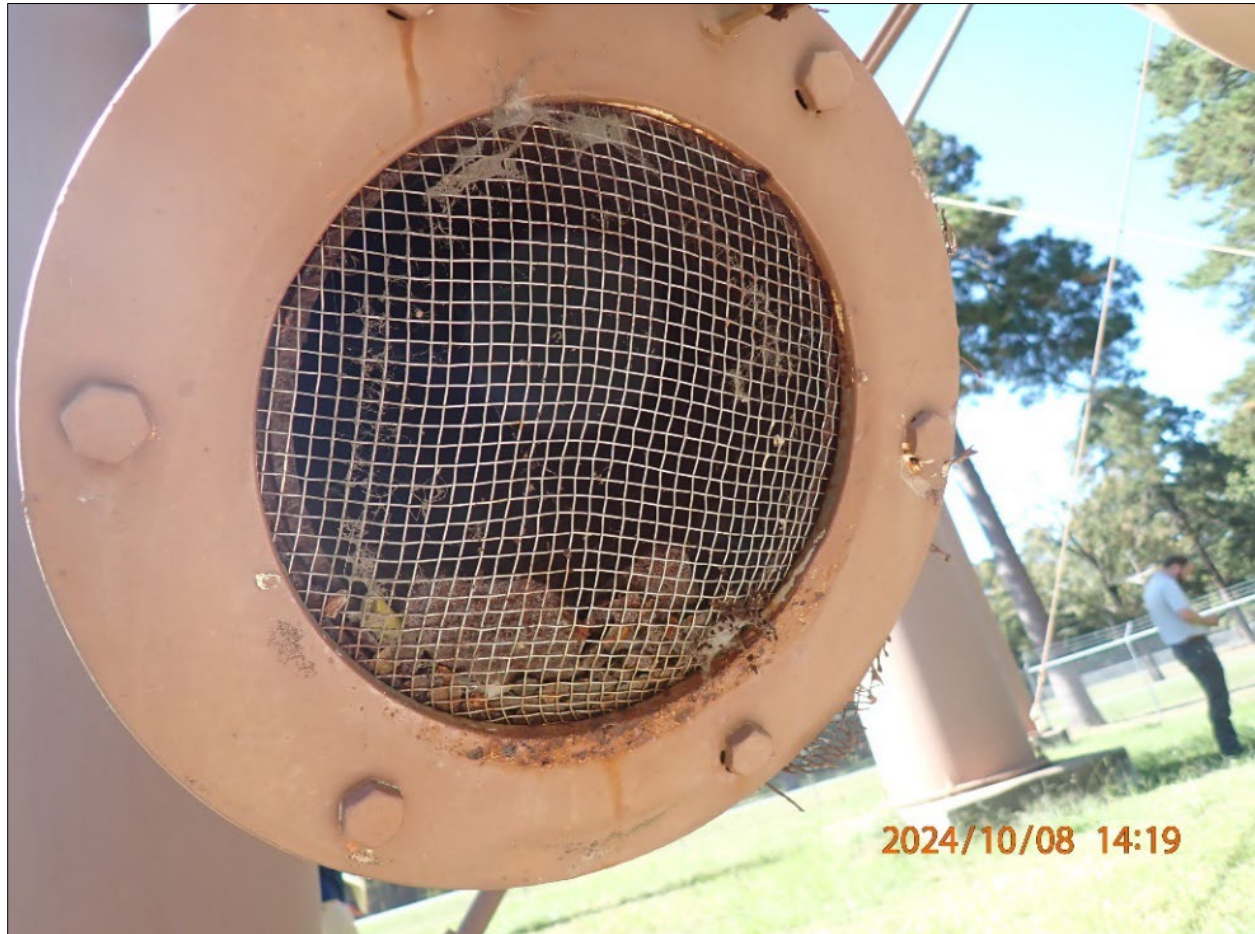
Photograph 6. East Side Elevated Storage Tower 10/08/2024 14:19 PA080251.JPG
