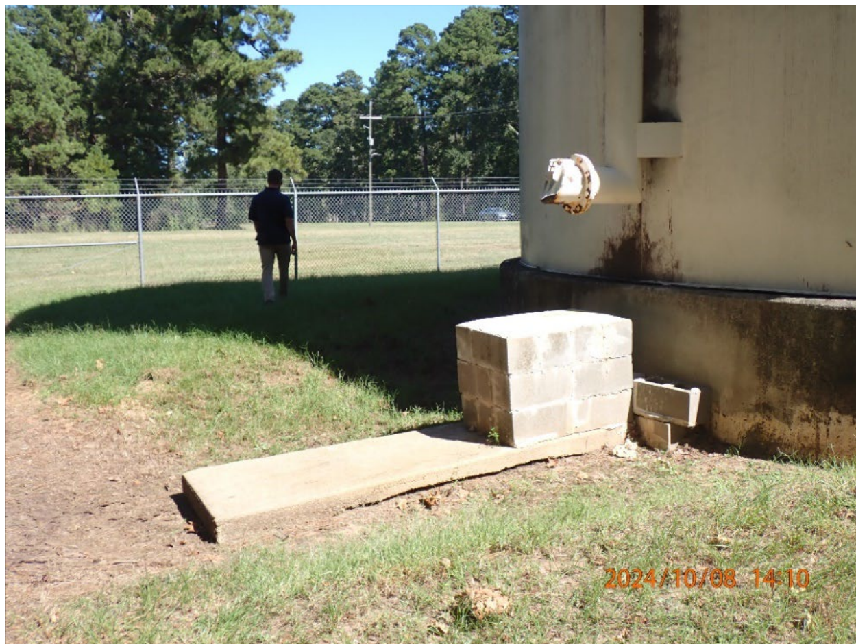
Photograph 8. East Housing Ground Storage Tank 10/08/2024 14:10 PA080245.JPG
