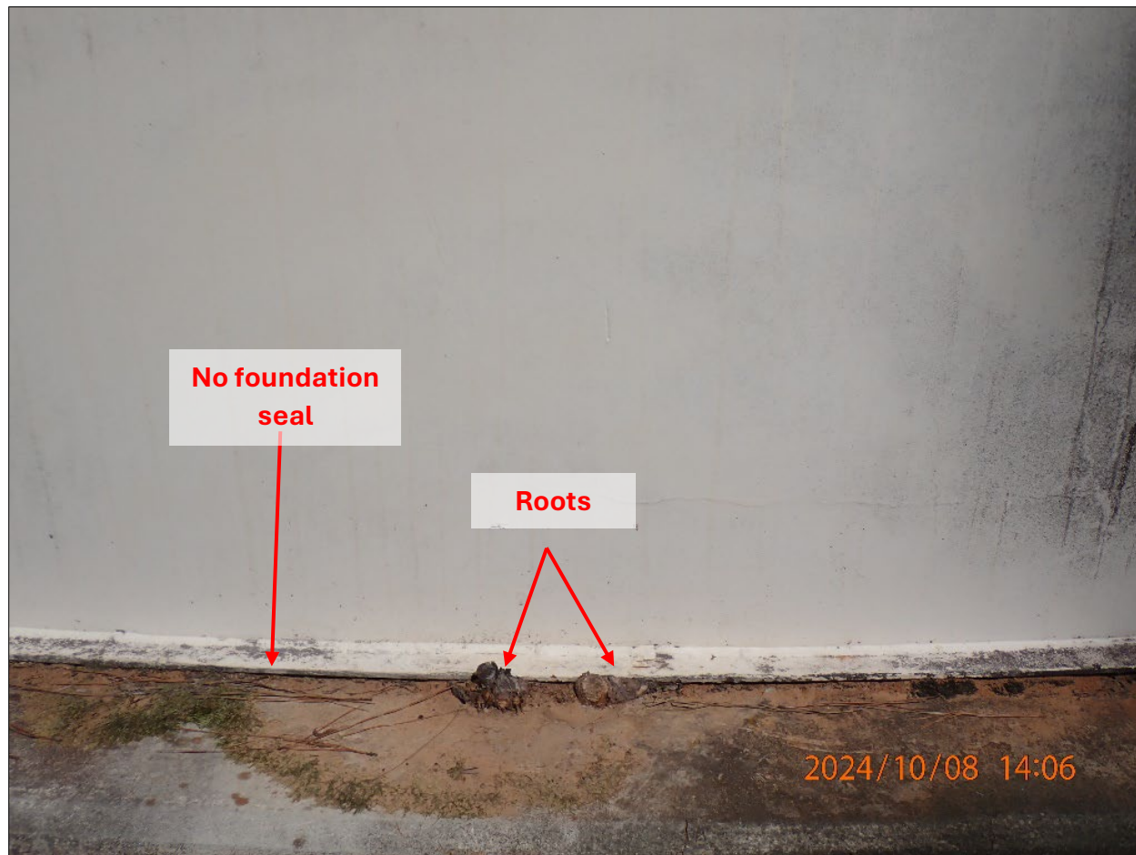
Photograph 10. East Housing Ground Storage Tank 10/08/2024 14:06 PA080239.JPG
