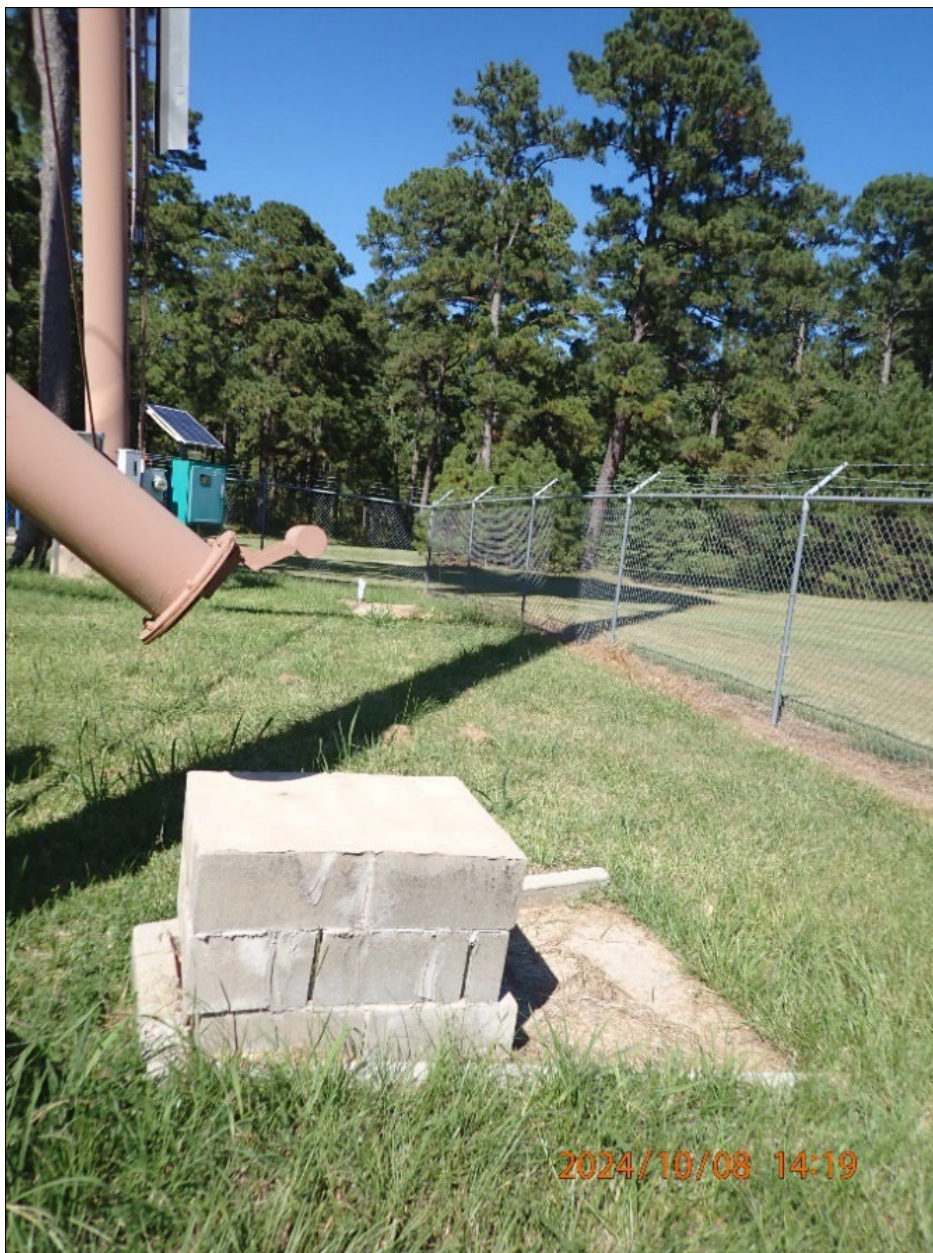
Photograph 9. East Side Elevated Storage Tower 10/08/2024 14:19 PA080250.JPG
