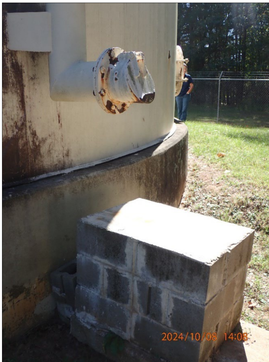
Photograph 7. East Housing Ground Storage Tank 10/08/2024 14:08 PA080244.JPG
