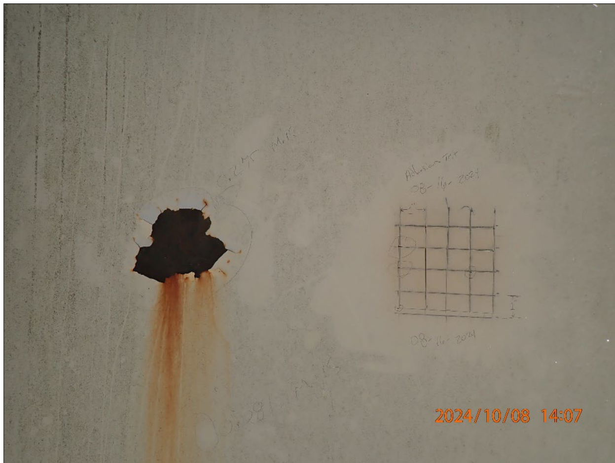
Photograph 12. East Housing Ground Storage Tank 10/08/2024 14:07 PA080241.JPG
