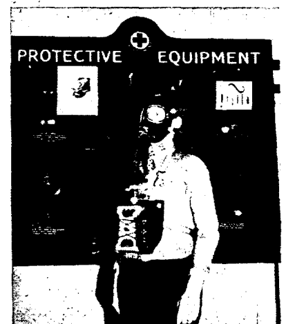
An all-service gas mask may be used in atmospheres where there is no oxygen deficiency.
