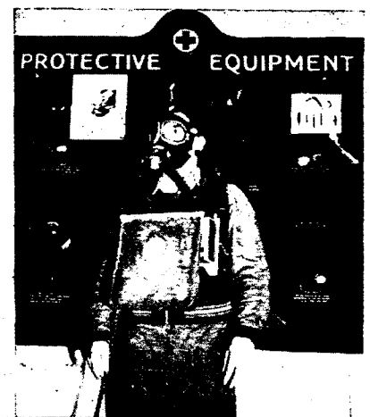
A shipyard worker wearing oxygen-breathing apparatus. In the background is a display of protective equipment, showing goggles, hard hats and safety shoes.
