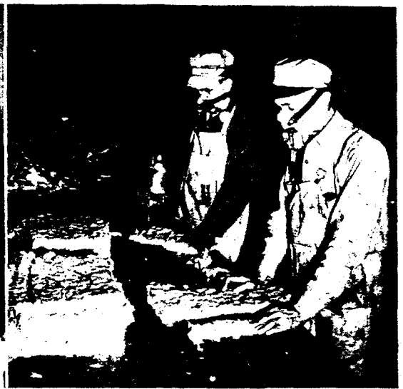
Men working with water-repellent asbestos insulation are equipped with dust respirators.
