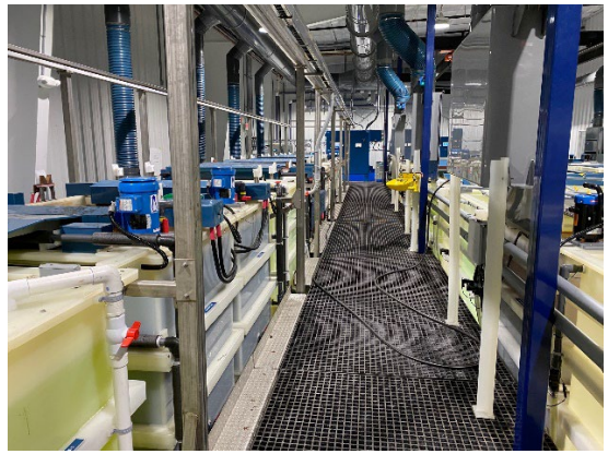
Photograph #8 – New Plating Building.
