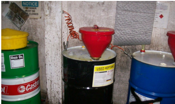
Photograph #1 – Used heptane container without “Hazardous Waste” and hazard indication label.
