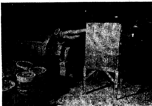
FIG. 6. LOCAL EXHAUST ON TUMBLERS FOR CAST CLEANING.
