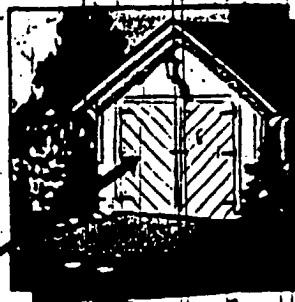
For the Garage
