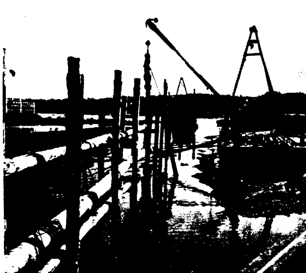
A section of the submarine line suspended by rope and chain falls before lowering into the water in sections of about 100 ft. long and already calked together
