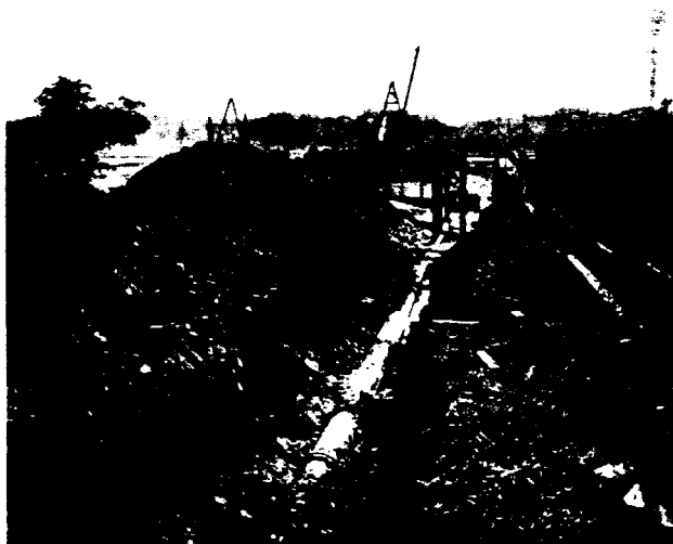
A section of the submarine line suspended by rope and chain falls before lowering into the water in sections of about 100 ft. long and already calked together
