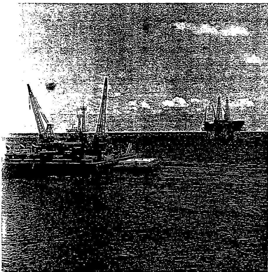
The Marine Pipeline Division set a new record when Lty Barge 29 installed a 12-inch pipeline in more than 1,000 feet of water in the Gulf of Mexico.
