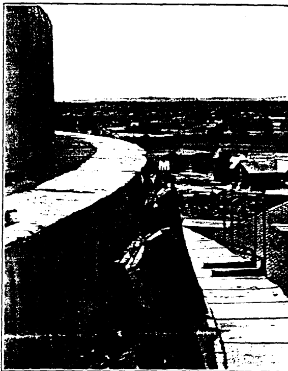
Partly completed job of recovering Rahway Reformatory dome with hard lead sheet for permanence and beauty.
