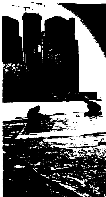
Lead burners for Allied Lead, Chicago, burn joints of lead sheets used to waterproof base of new $2 million fountain in downtown Detroit.
