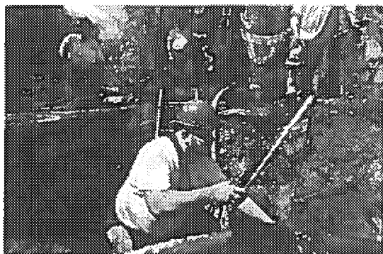
The Pittsburgh Water and Sewer Authority's Ryan Hungerman worked to repair a broken lead water line at a home last week. PHOTO: JUSTIN MERRIMAN FOR THE WALL STREET JOURNAL
