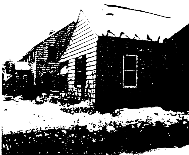
A typical installation of lead sheathed heating cable for snow melting purposes. The saw tooth pattern provides channels for complete drainage.
