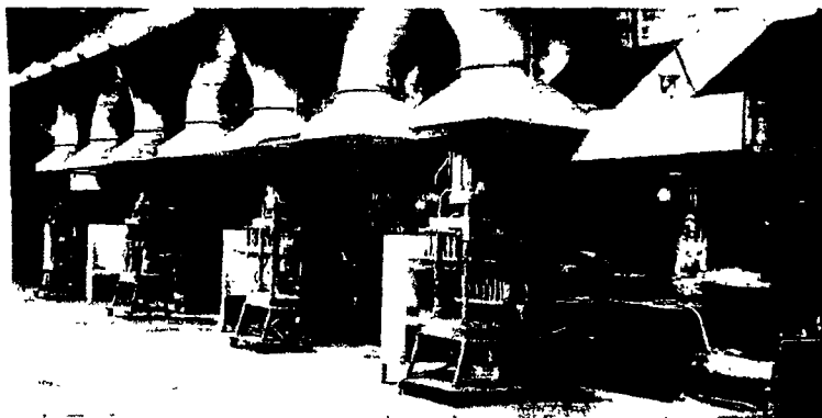
Figure 7. In this foundry, local exhaust hoods are installed over each station having a shell-molding machine and glue press. Adequate make-up air is supplied from ventilating duct situated between molding machines and presses. (Courtesy American Foundrymen's Society)
