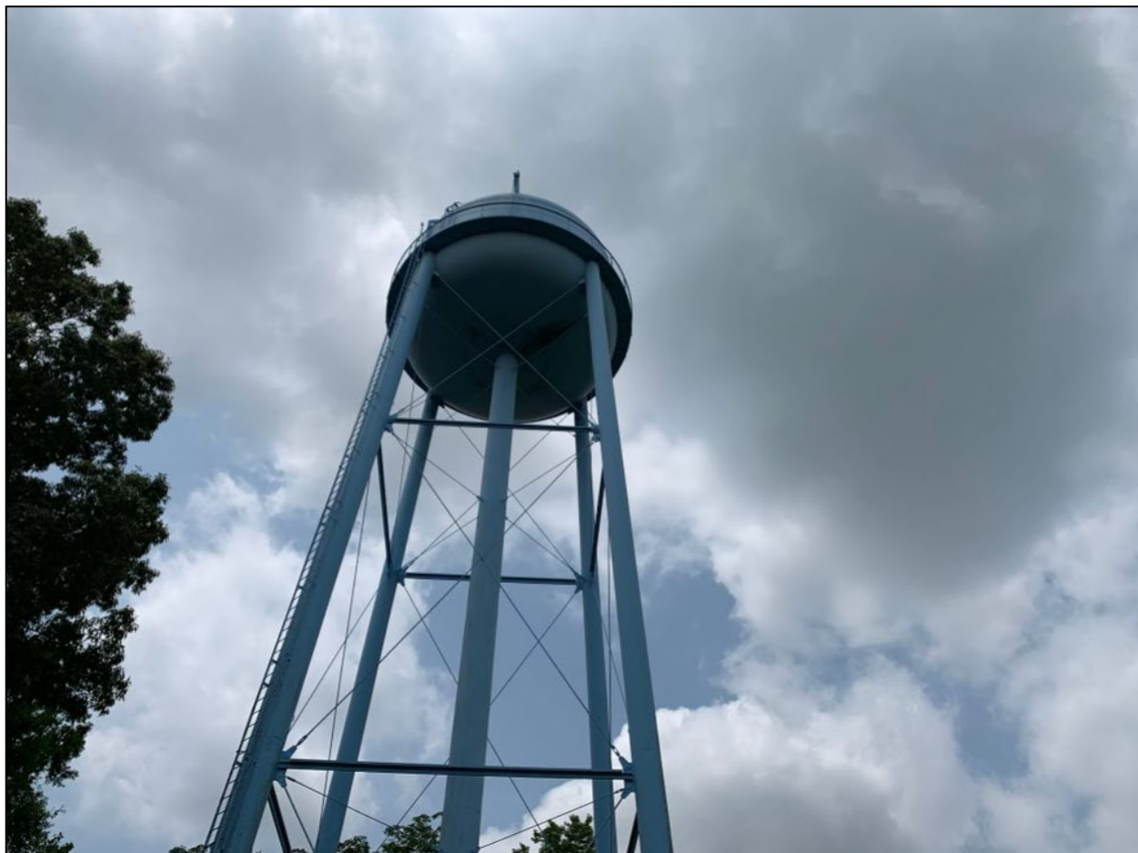
Photograph 16. West Point Water Tank View of the West Point Water Tank. The tank is an elevated, 100,000-gallon storage tank.
