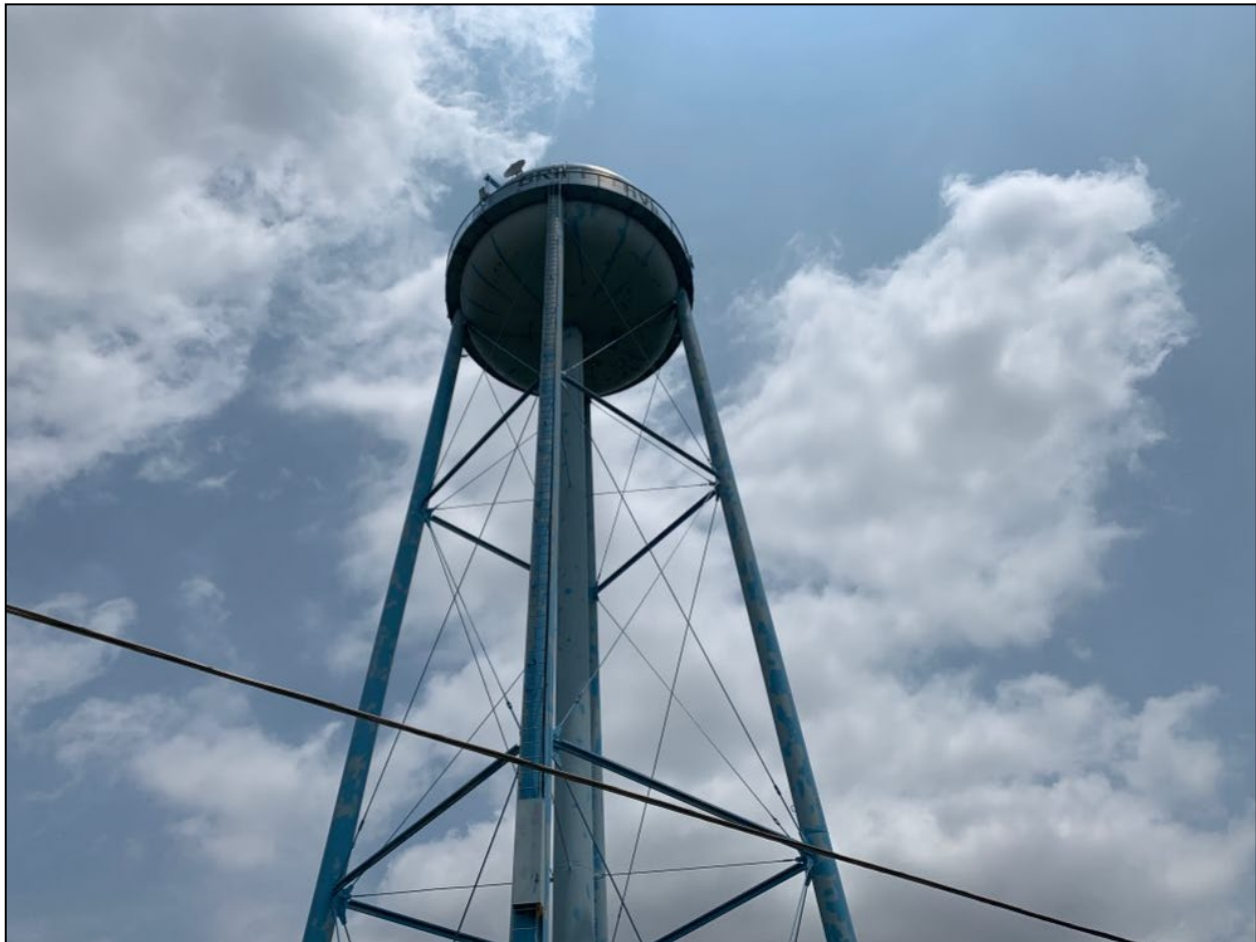
Photograph 23. Griffithville Water Tank View of the Griffithville Water Tank. The tank is an elevated, 100,000-gallon storage tank.
