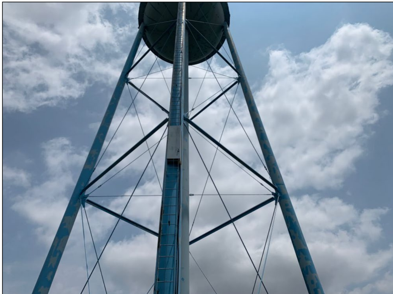
Photograph 27. Security Ladder, Griffithville Water Tank View of the security ladder and ladder shield at the Griffithville Water Tank. The ladder shield was locked, and the bottom rungs of the ladder were removed.
