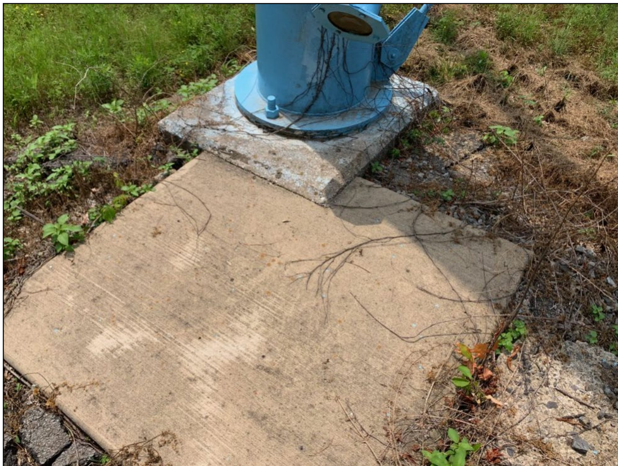
Photograph 25. Concrete Splash Pad, Griffithville Water Tank View of the concrete splash pad beneath the end of the Griffithville Water Tank overflow pipe.
