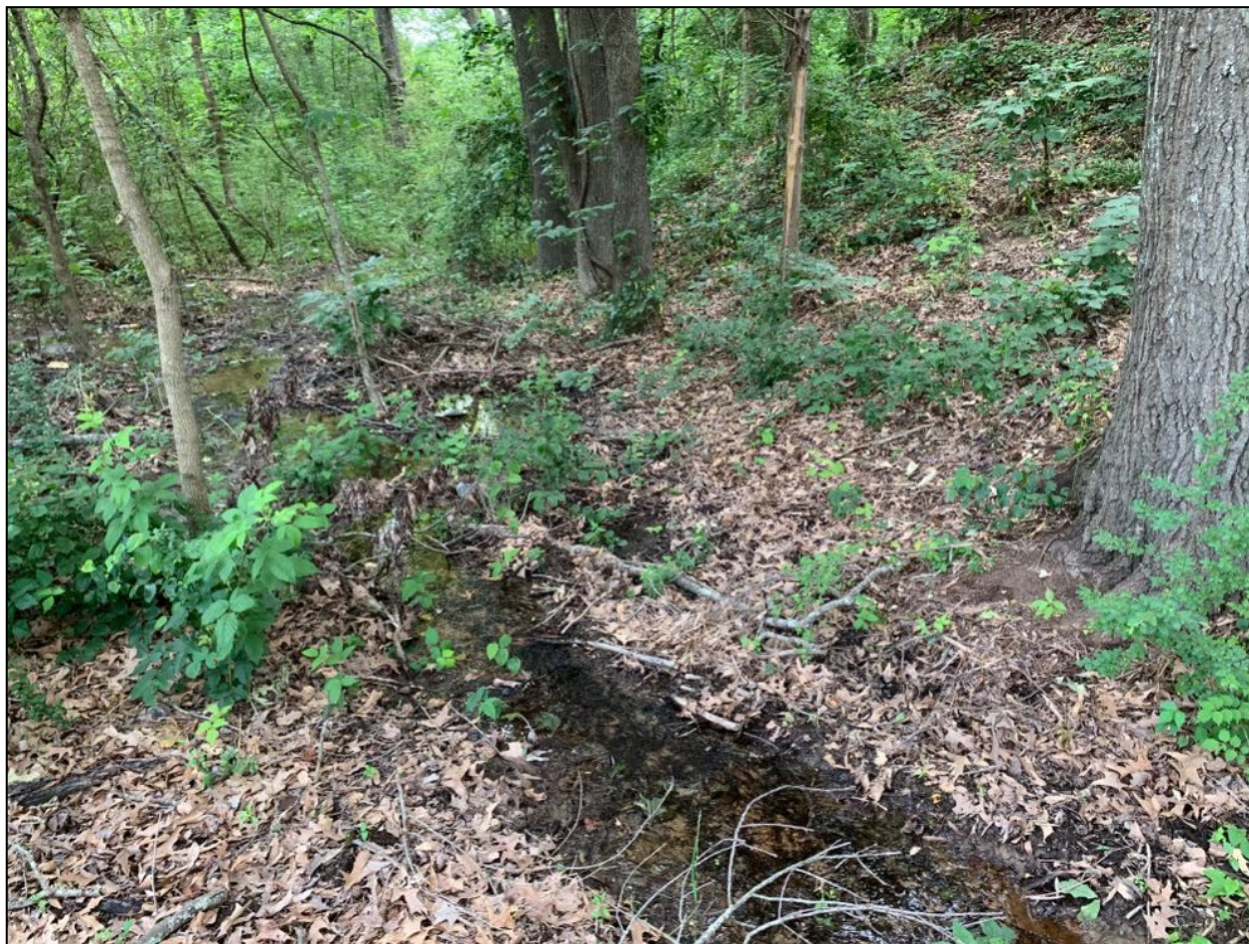
Photograph 12. Water Leak, Master Meter #3 View of the water leak upstream of Master Meter #3 running downhill away from the meter vault.
