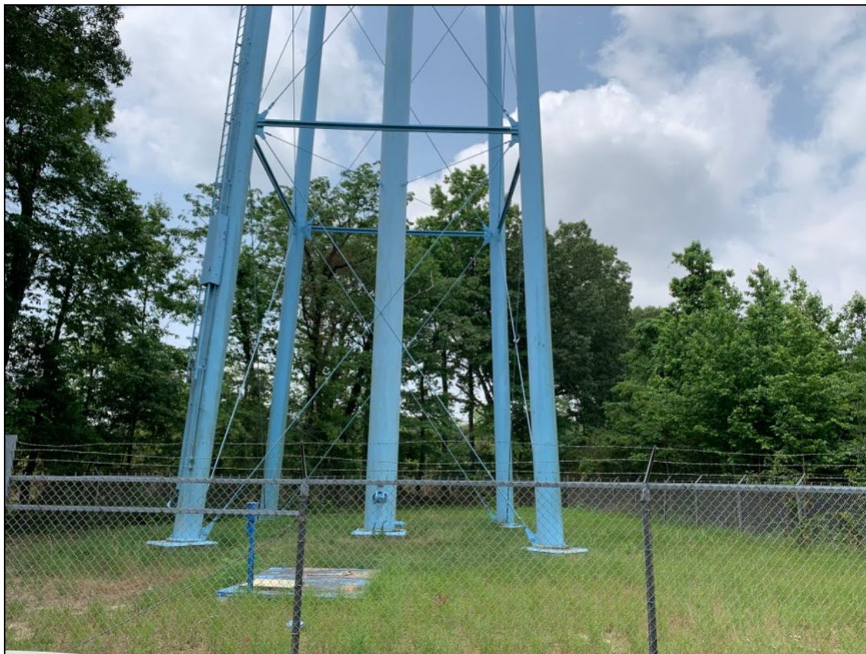
Photograph 17. Perimeter Fence, West Point Water Tank View of the locked security fence that surrounded the West Point Water Tank. The fence was equipped with barbed wire.
