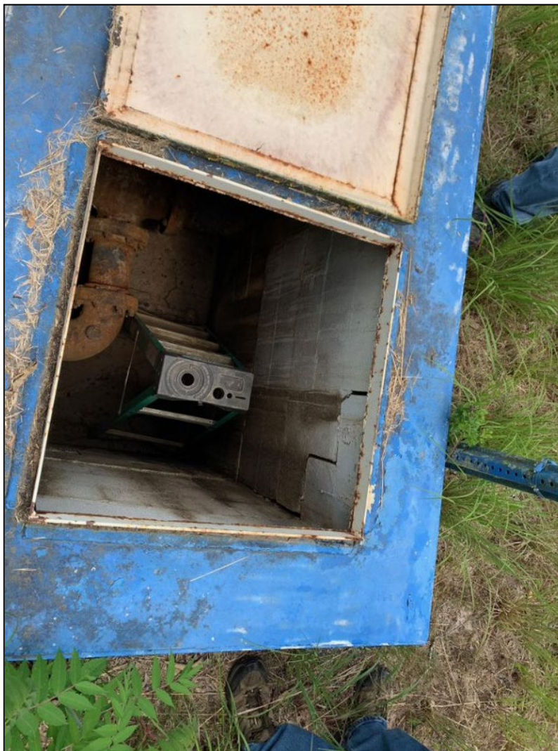
Photograph 22. Valve Vault, West Point Water Tank View of the inside of the valve vault located next to the West Point Water Tank. The vault contained an altitude valve used to regulate the water level inside of the tank. [REDACTED]
