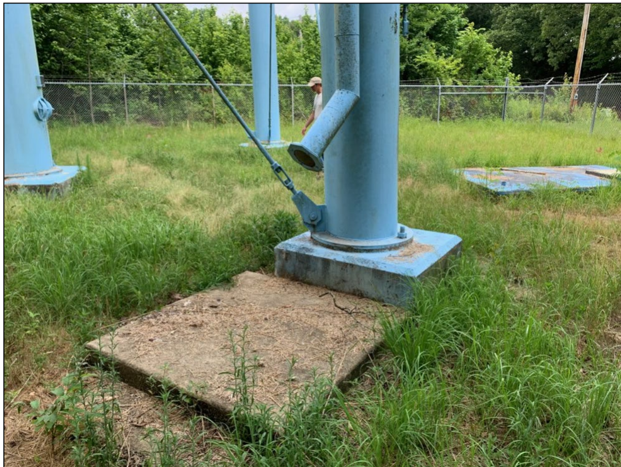
Photograph 19. Concrete Splash Pad, West Point Water Tank View of the end of the overflow pipe at the West Point Water Tank. The pipe ended over a concrete splash pad and contained a 24-inch mesh screen covering the opening.
