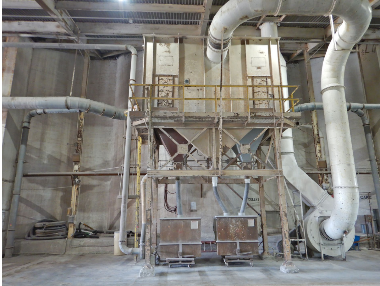
Photo 8 – Silo common dust collector
