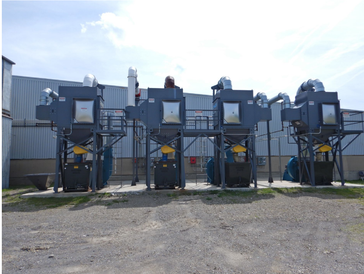
Photo 17 – Lucor dust collector
