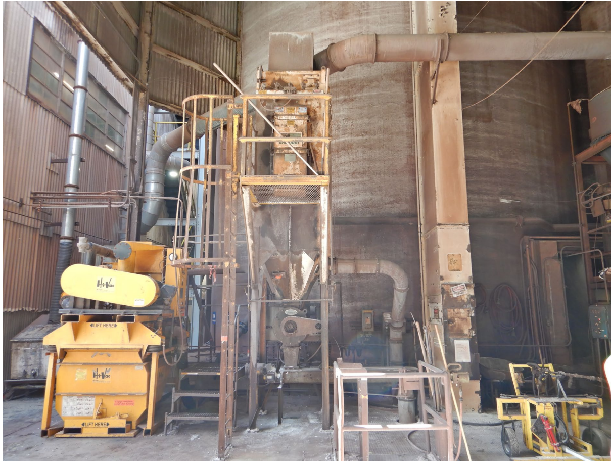
Photo 7 – Soda Ash dust collector
