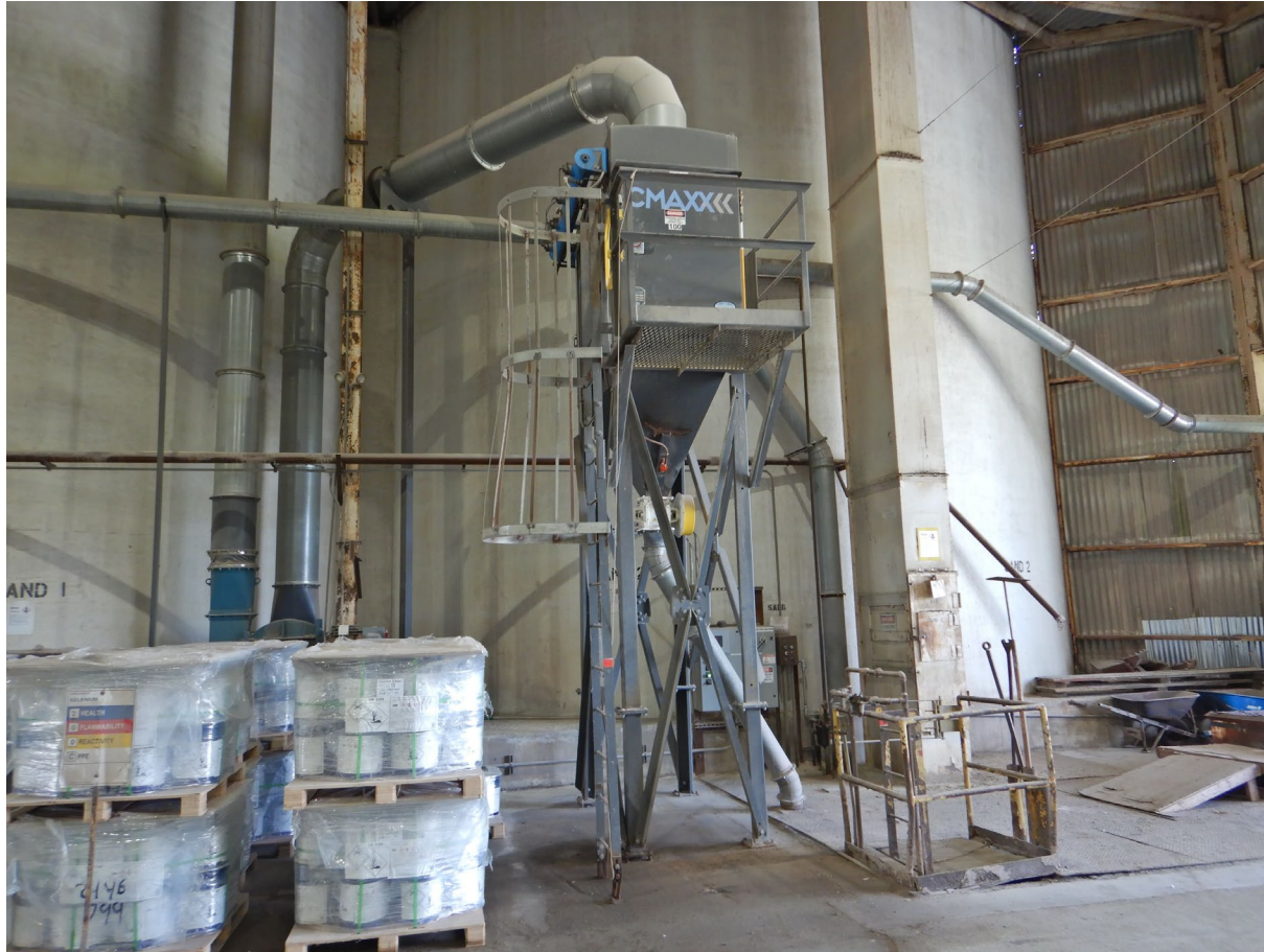
Photo 9 – Sand silo dust collector
