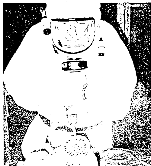
Fig. 4 (top): Removing an after service asbestos-containing gasket from a pipe flange by hand-scraping.
