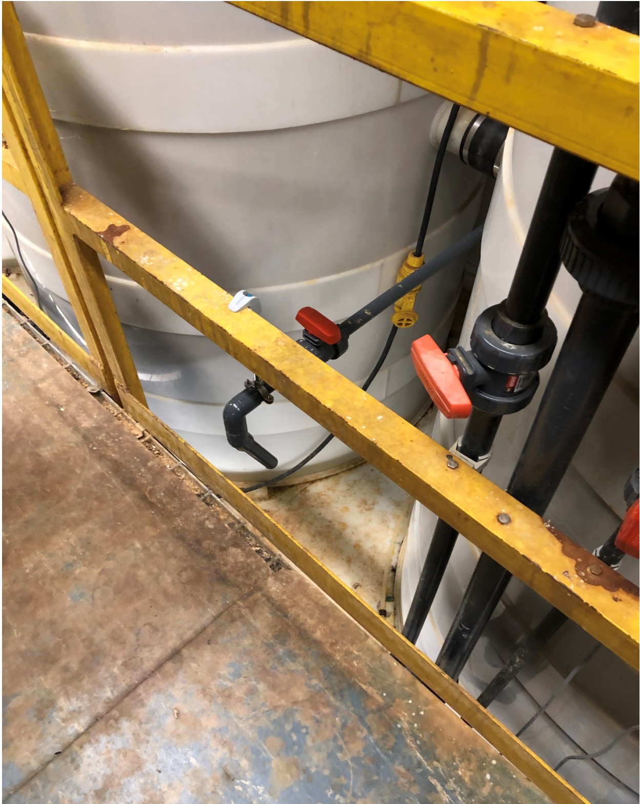
Photo #1: View of the sample tap at Tank TR-2 where the cyanide sample was collected.
