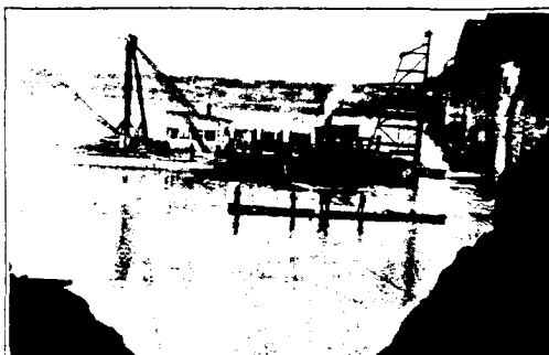
Laying high-voltage submarine cable across the Mississippi River at St. Louis
