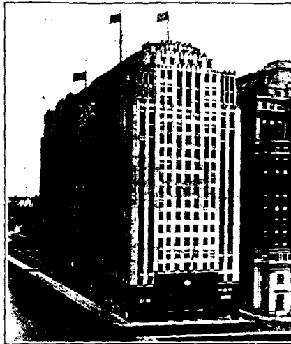
COURTESY PENNSYLVANIA R. R. CO. NEW OFFICE BUILDING and suburban station of the Pennsylvania Railroad near the site of present Broad Street Station Graham, Anderson, Probst and White, Architects
