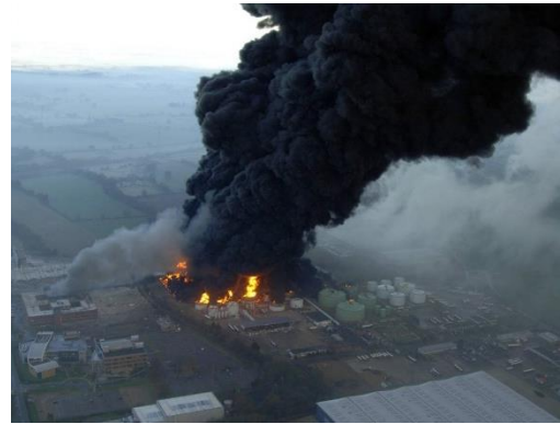
Figure 3 - Buncefield fire, England (2005). Caused by instrumentation failure.
