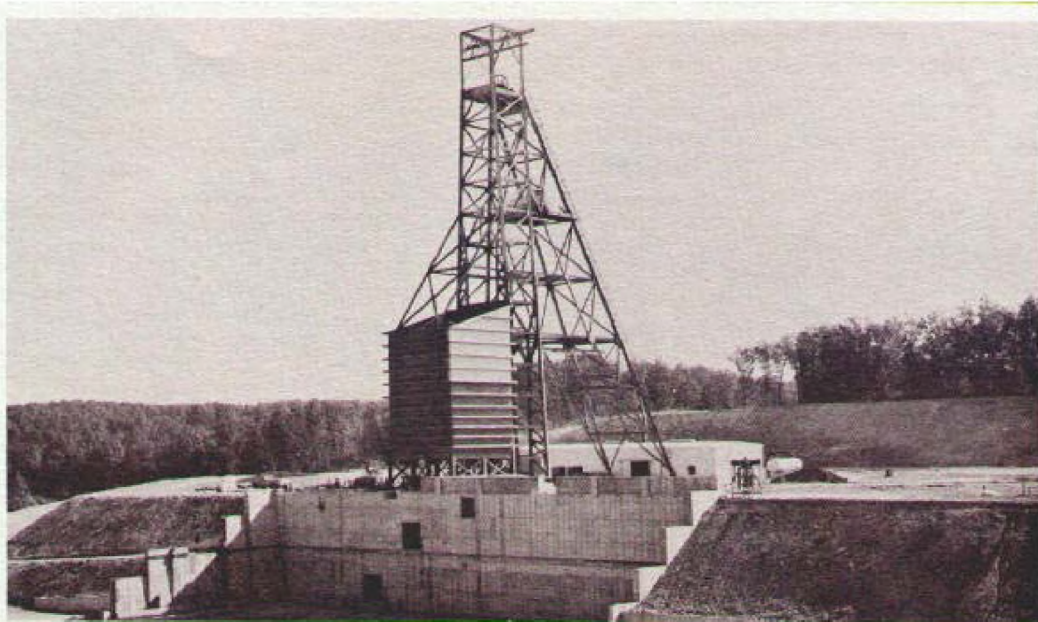
BRUSHY CREEK PLANT SITE Completion date set for 1973.
