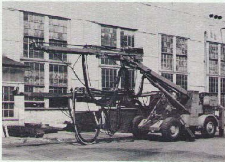
Jumbo with two rotary percussion drills.
