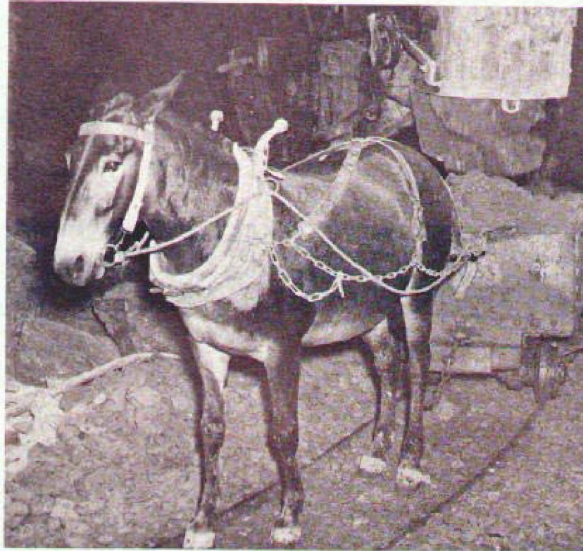
SCENE UNDERGROUND DURING THE EARLY THIRTIES Mules were used to pull loaded mine cars from heading to main line.
