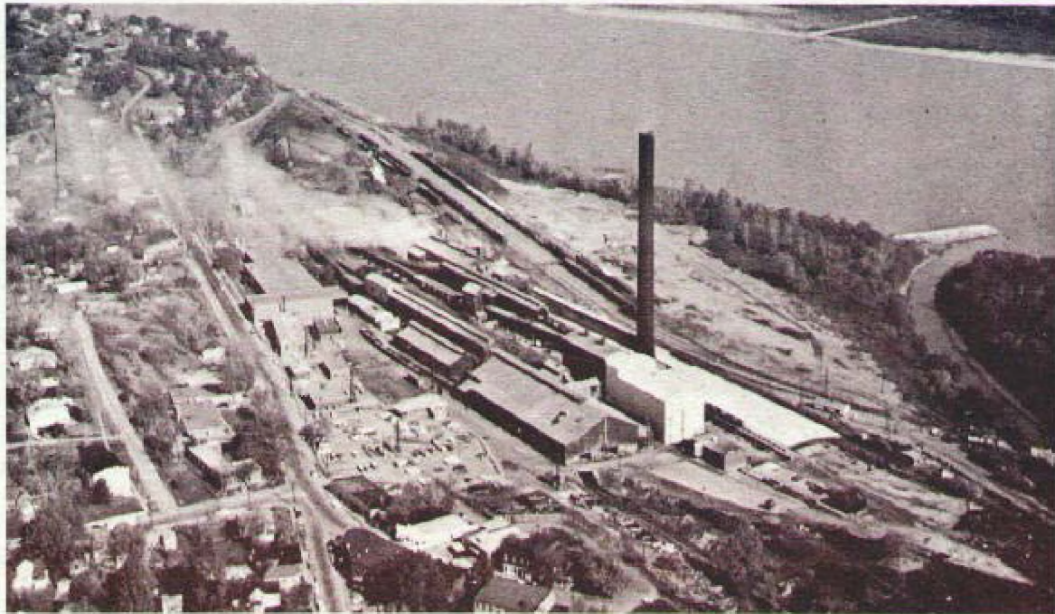
HERCULANEUM SMELTER IN, JEFFERSON COUNTY MISSOURI Processes concentrates from St. Joe operations.
