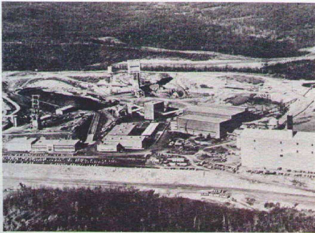
Meramec Mining Company in Washington County, Missouri Began production of iron pellets in 1964.
