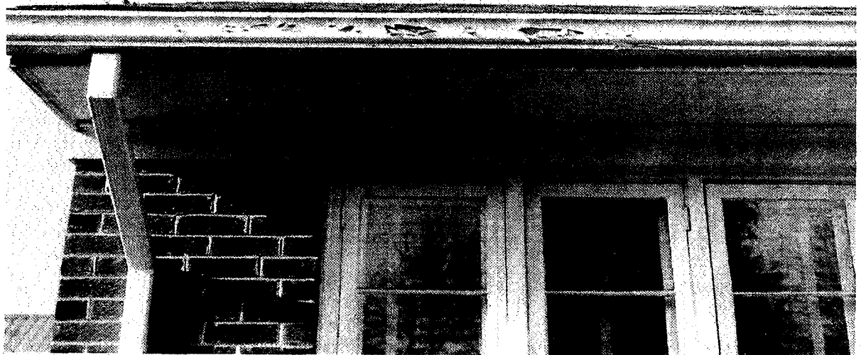
Figure 95. Peeling from Galvanized Gutters.
