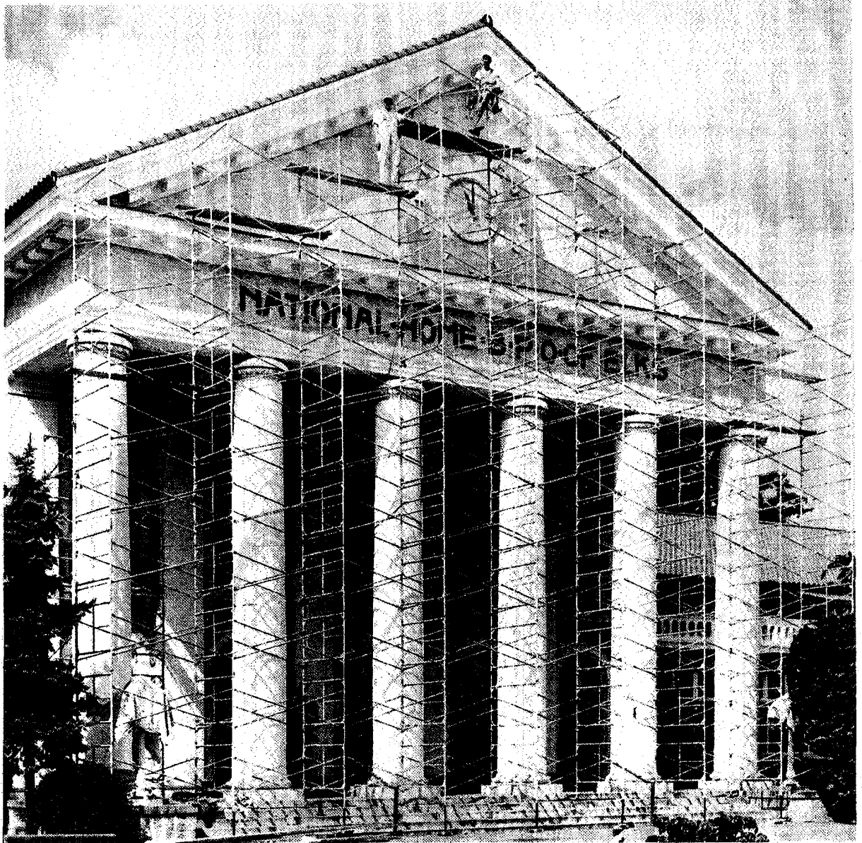
Figure 19. Pipe Scaffolding.
