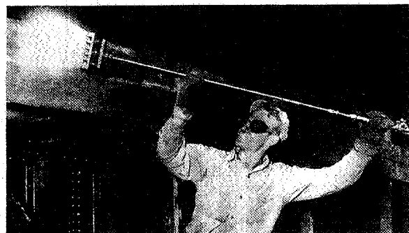
Figure 42. Flame Cleaning.
