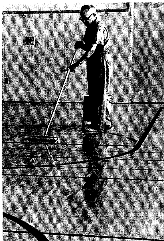
Figure 119. Applying Clear Floor Finishes.
