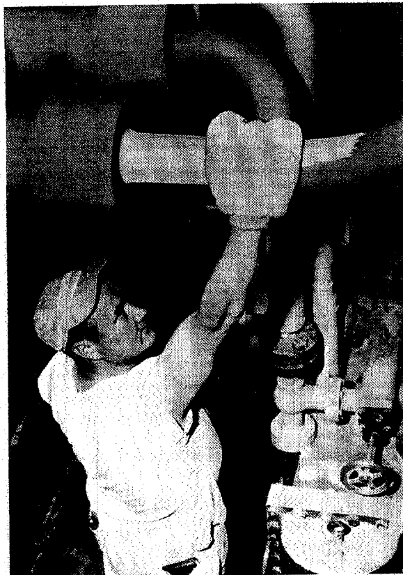
Figure 76. Paint Mitt in Use.
