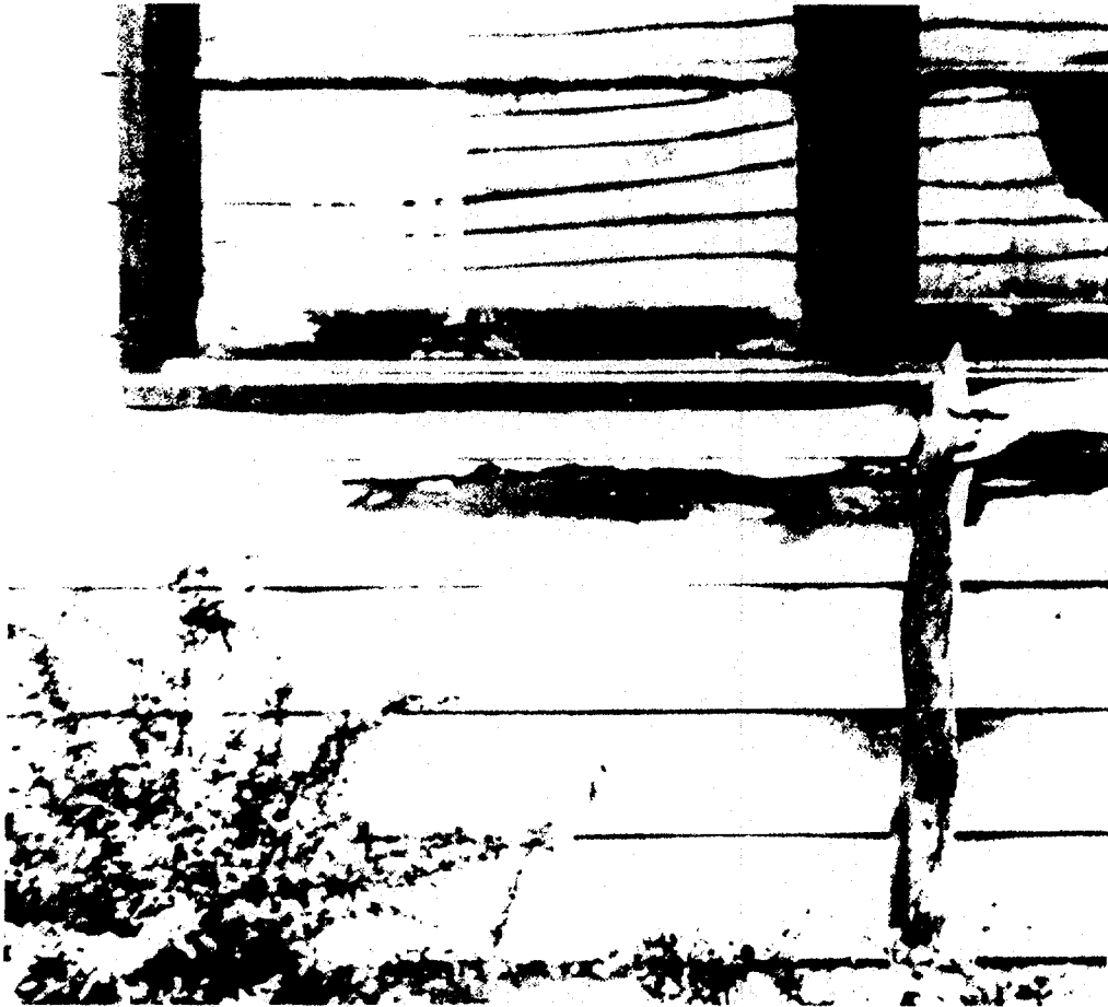
Figure 111. Moisture Peeling Caused by Contact with Ground.
