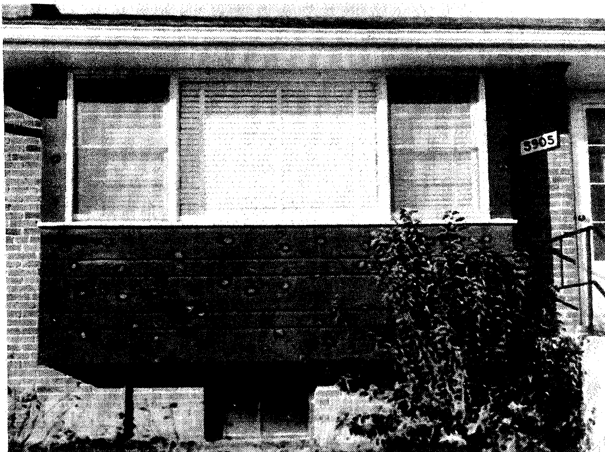
Figure 93. Bleeding Around Knots.
