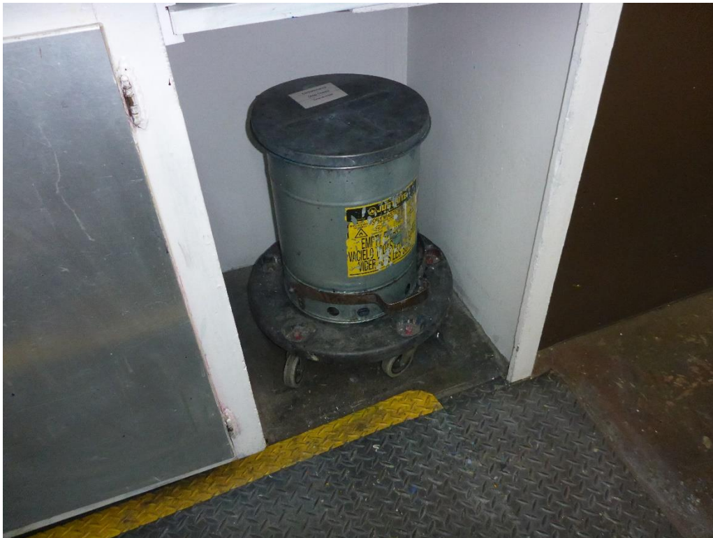
Photo 10: One 5-gallon flip-top container for accumulating solvent contaminated wipes in the Ink Lab. The container was not labeled “excluded solvent contaminated wipes.”
